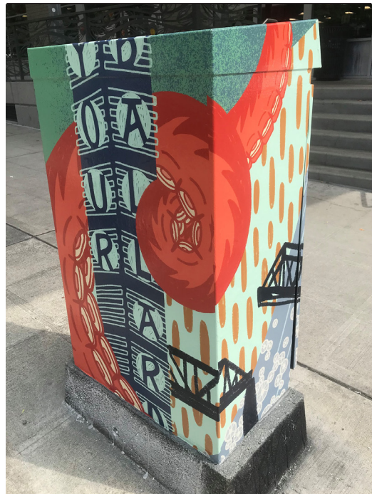
WRAPPED UTILITY BOX ON NW 57TH ST & 24TH AVE NW
