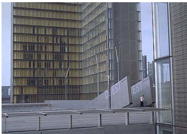
(Fig 3.3): The new Bibliotheque National. The transparent towers protected by wooden shutters.
