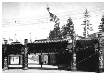
Railroad overpass. (UWSC AYP631)
