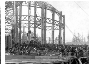
Constructing the U.S. Govt. Building. (UWSC AYP498)
