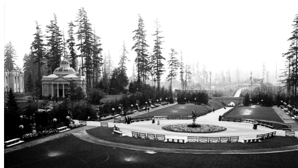
Looking south across Rainier Circle.
