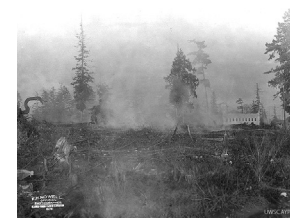
Clearing the site for the U.S. Govt. Building. (UWSC AYP489)
