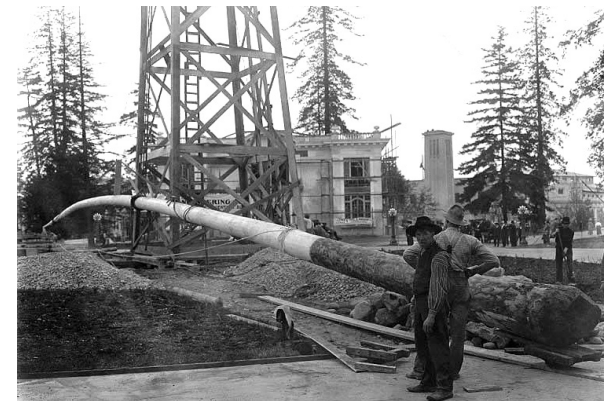
The installation of the flagpole in Dome Circle. (UWSC AYP490)
