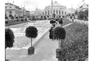
Cascade Court looking north. (UWSC AYP216)
