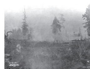
Clearing the site for the U.S. Govt. Building. (UWSC AYP489)
