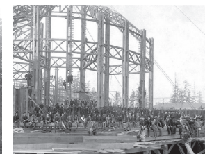
Constructing the U.S. Govt. Building. (UWSC AYP498)
