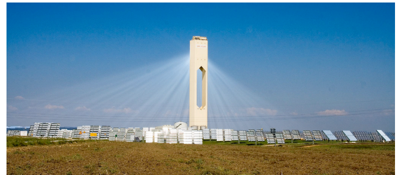
A solar thermal facility 1
