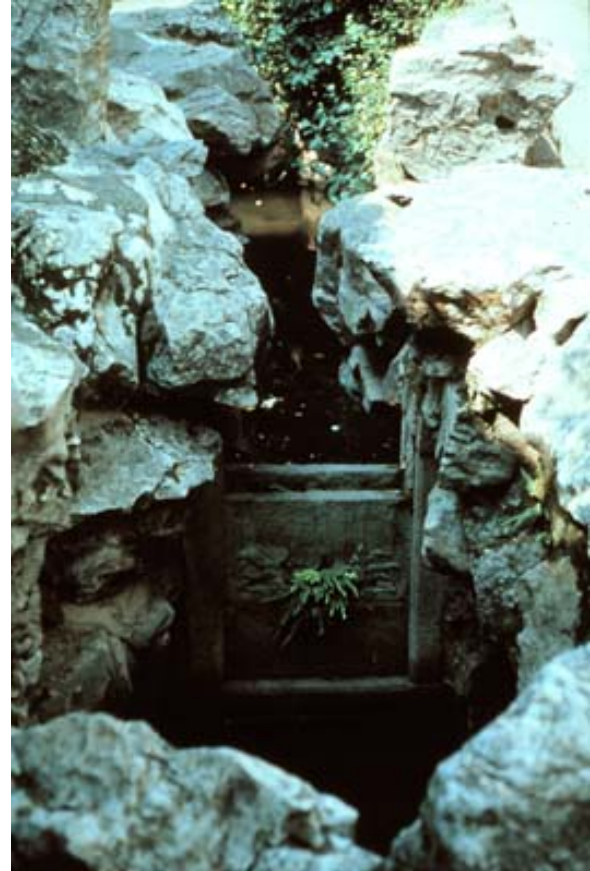
Sluice gate at pond "source"
