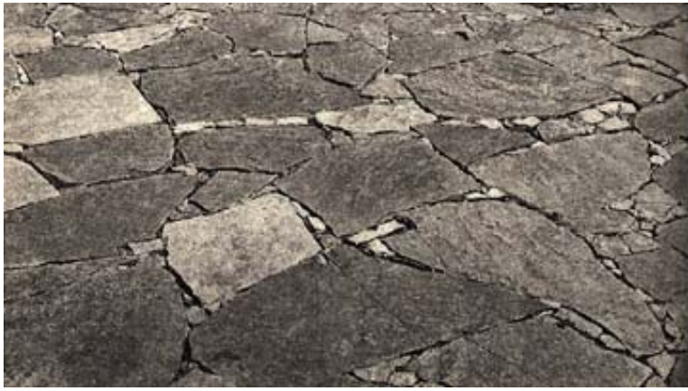
SOURCE: Liu Dunzhen, ed., Suzhou gudian yuanlin (Nanjing: Zhongguo jianzhu gongye chubanshe, 1979), p. . Cracked ice tiling, Garden of the Master of Nets, Suzhou.
