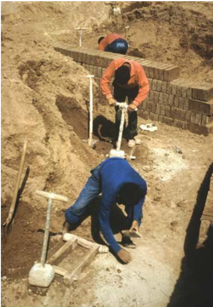
Earth being used to fill frames for bricks in Gansu province
