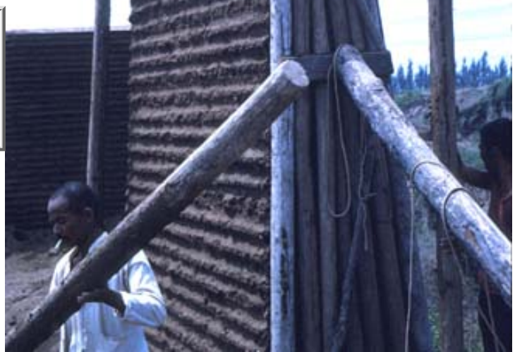
Building an earthen wall, Xi'an area, Shaanxi Province
