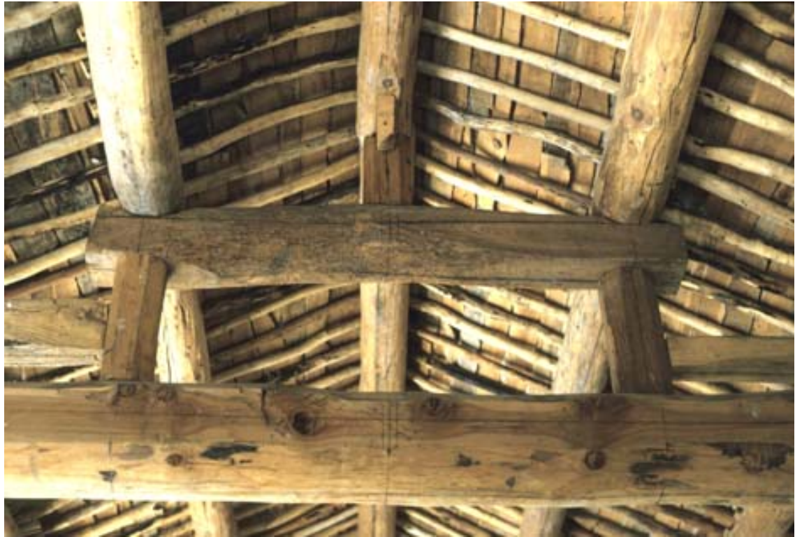
Pillars-and-beams wooden roof support system, from a building in the Beijing area
