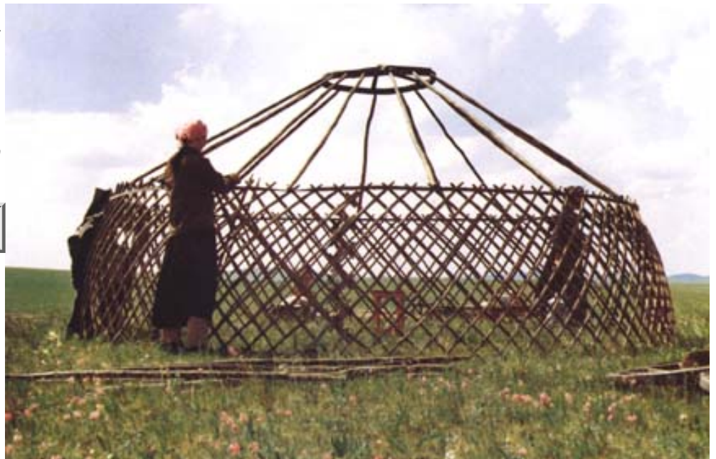
Building a yurt in Inner Mongolia
