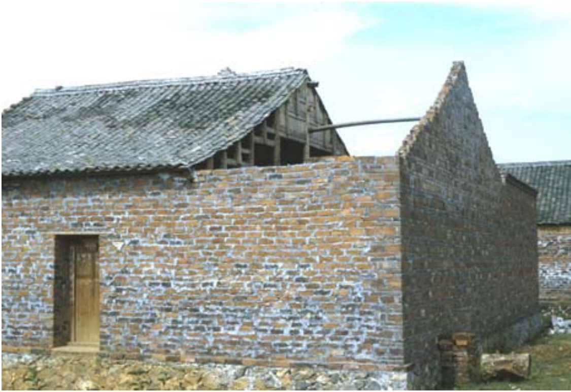
Brick house with timber structure exposed in Guangxi province
