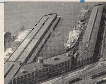
Stacey-Lander Terminal at the Port of Seattle offers 2,186 ft. of berthing space, with modern truck, rail, and elevator facilities.
