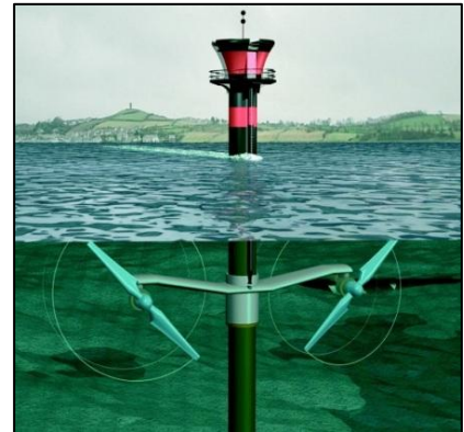
b. Marine Current Turbine SeaGen MHK turbine
