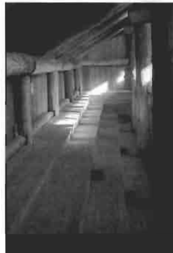
PHOTO 5. Interior of the main room: upper bleacher seating area.
