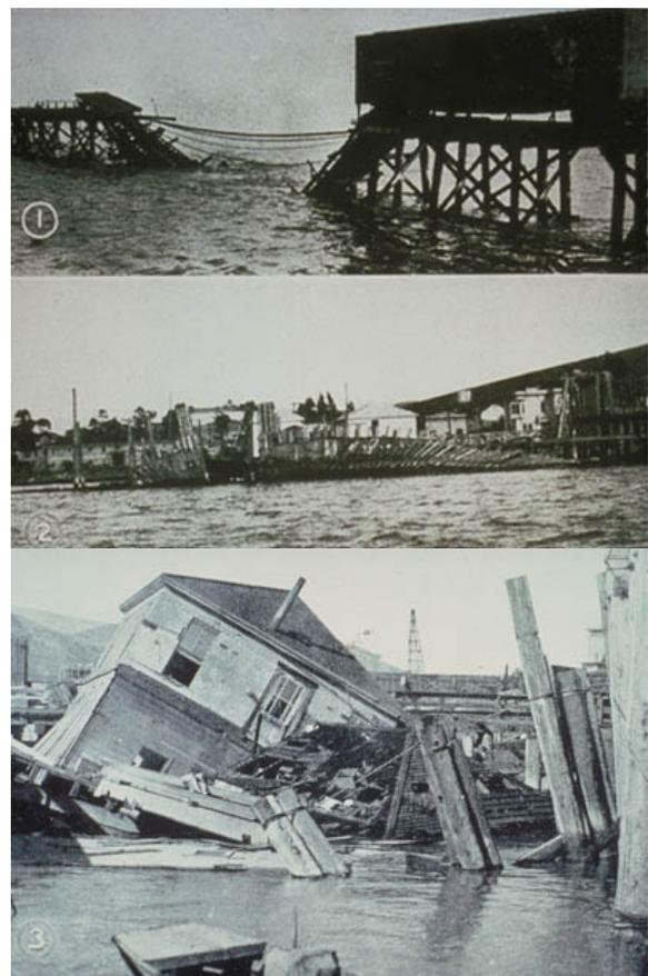
Figure 7: After its introduction to San Francisco Bay in 1913, the shipworm resulted in an estimated \$3.1 billion in damage to wooden structures between 1919 and 1921.
