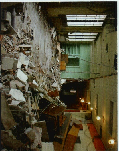
Construction funding for the renovation of Johnson Hall was approved by the state in the 2003-2005 capital budget.
