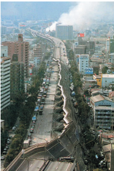
Damage from Kobe earthquake http://
