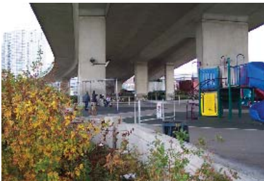
Play space, basketball courts and a greenway link are provided under the Cambie Bridge on the Vancouver Waterfront (Photo: Nathan Brightbill).
