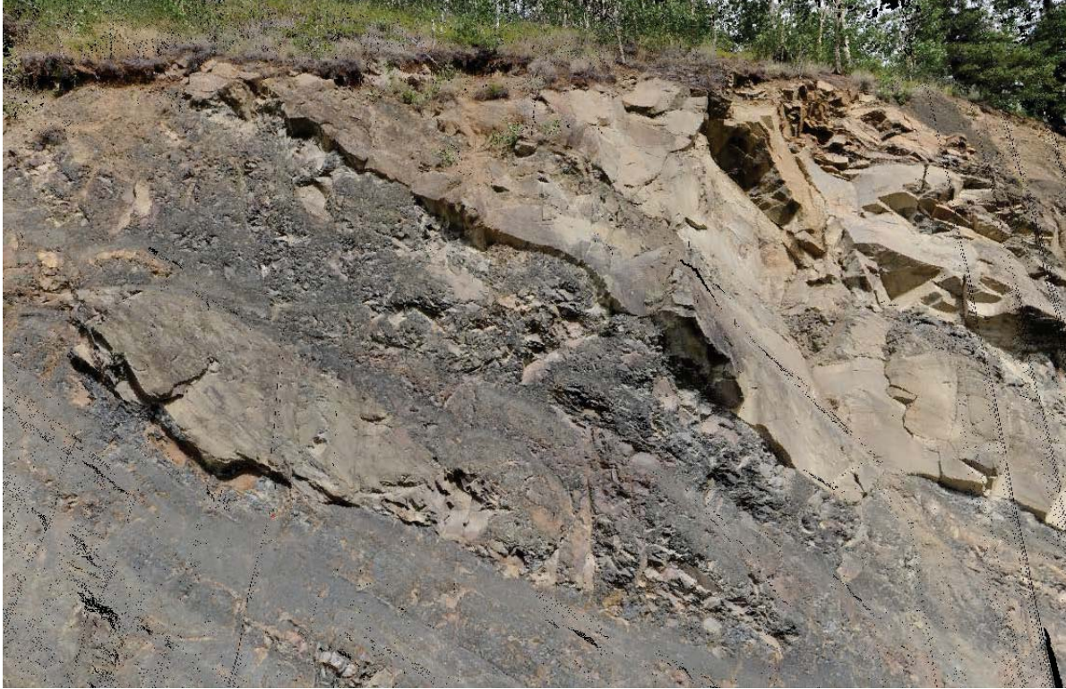
Figure 4.6 Close-up of the RGB colored point cloud at the Glitter Gulch project site, highlighting unstable rocks.
