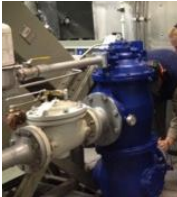
Figure 1.3 Self-cleaning filter installed on M/V Chetzemoka
