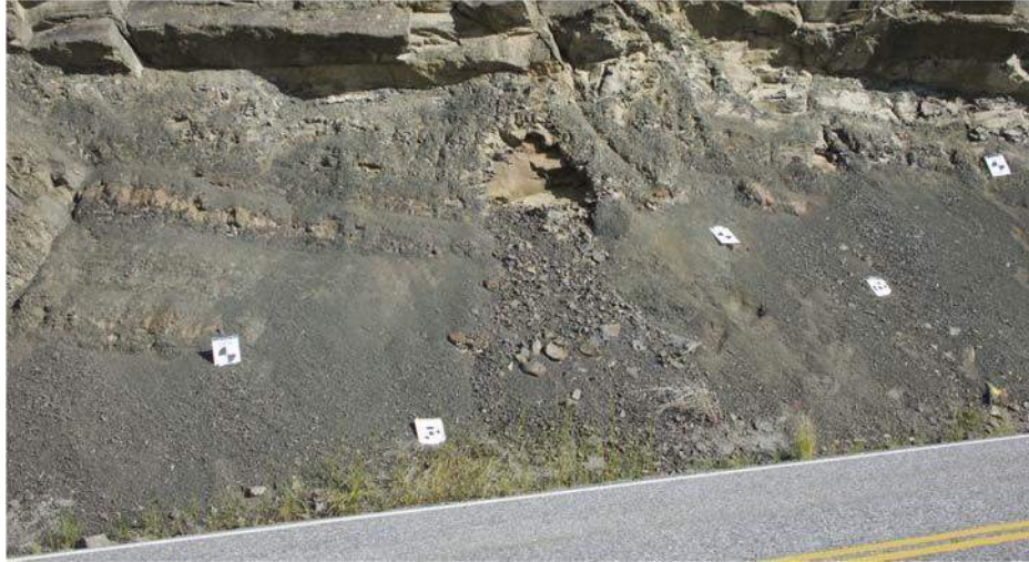
Figure 4.3 - Example of survey targets placed on the slope
