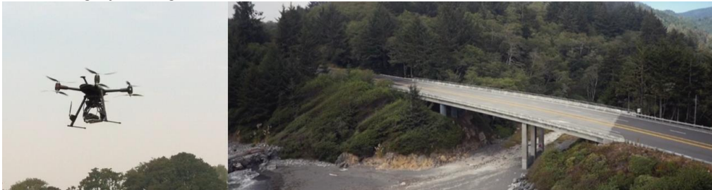
Example of imagery of a bridge acquired from an Aerialtronics octocopter (left). The image shown here was acquired at a relatively large stand-off distance and flying height to capture the entire deck. For high-resolution inspection work, the UAV can be operated at a shorter, fixed stand-off distance and/or a larger focal length camera can be utilized.
