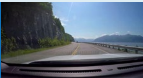
Passing zone on a compound curve (Seward Highway along Turnagain Arm, Alaska) illustrated how environmental and geometric conditions affect available and usable sight distance.
