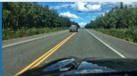
A motorist passes another vehicle in a “double yellow” striped area situated on a long vertical curve on the Parks Highway (near Cantwell, Alaska).
