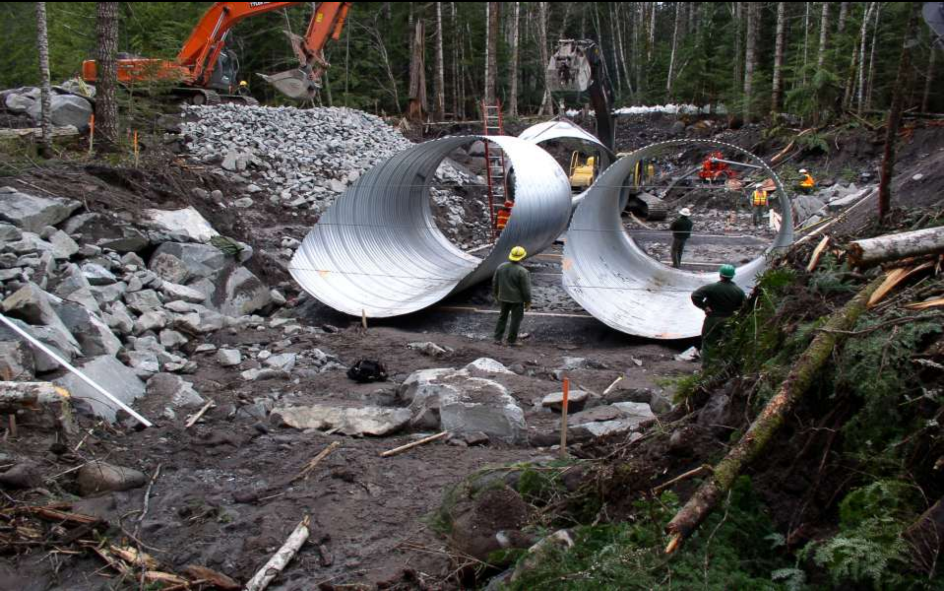
Culvert placement in Nisqually Road at Kautz Creek
