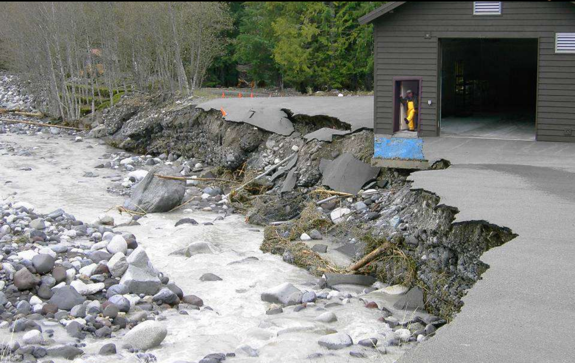
The park's Emergency Operations Center was undermined by the river.
