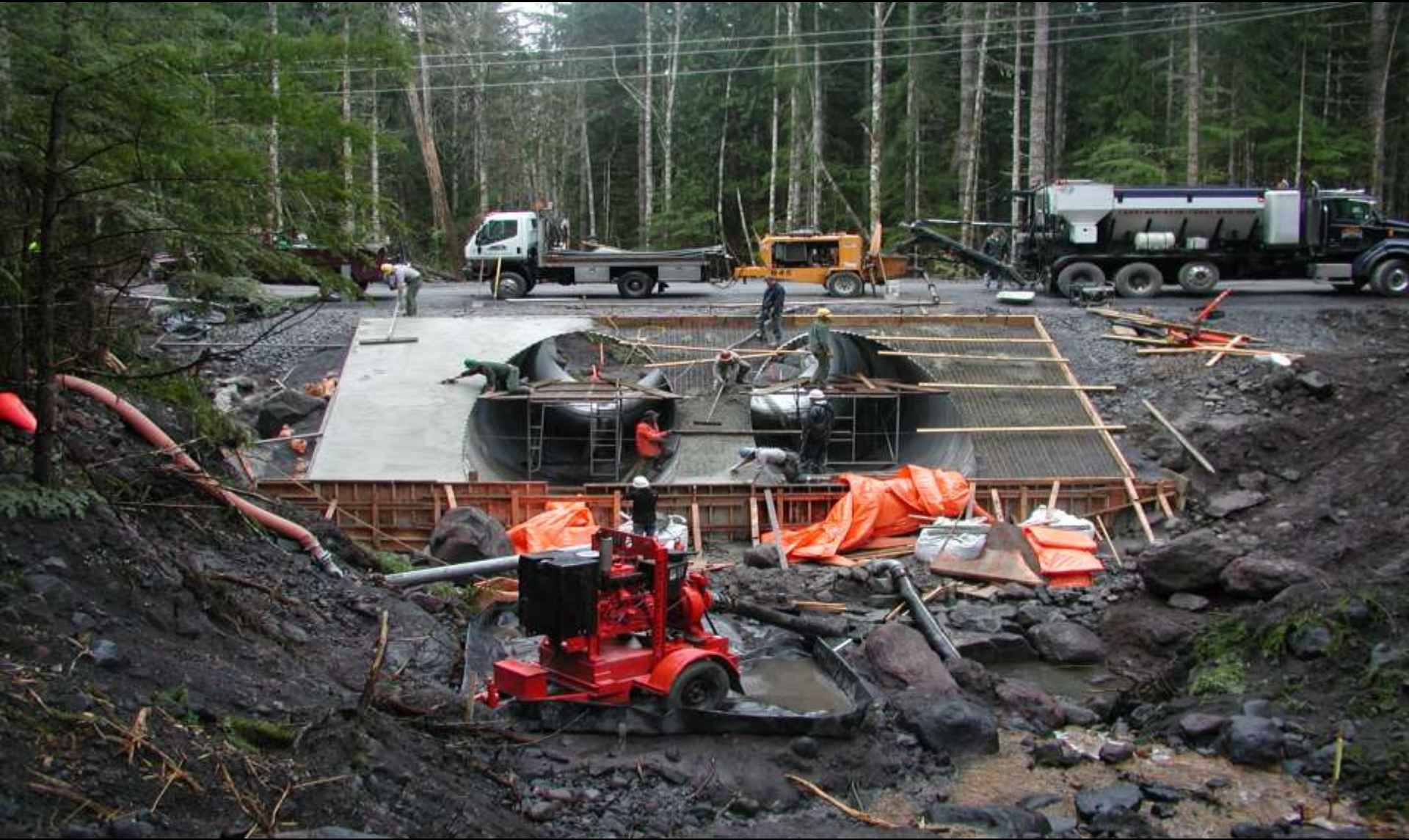
Finishing cement work on the up hill side of the Kautz culverts
