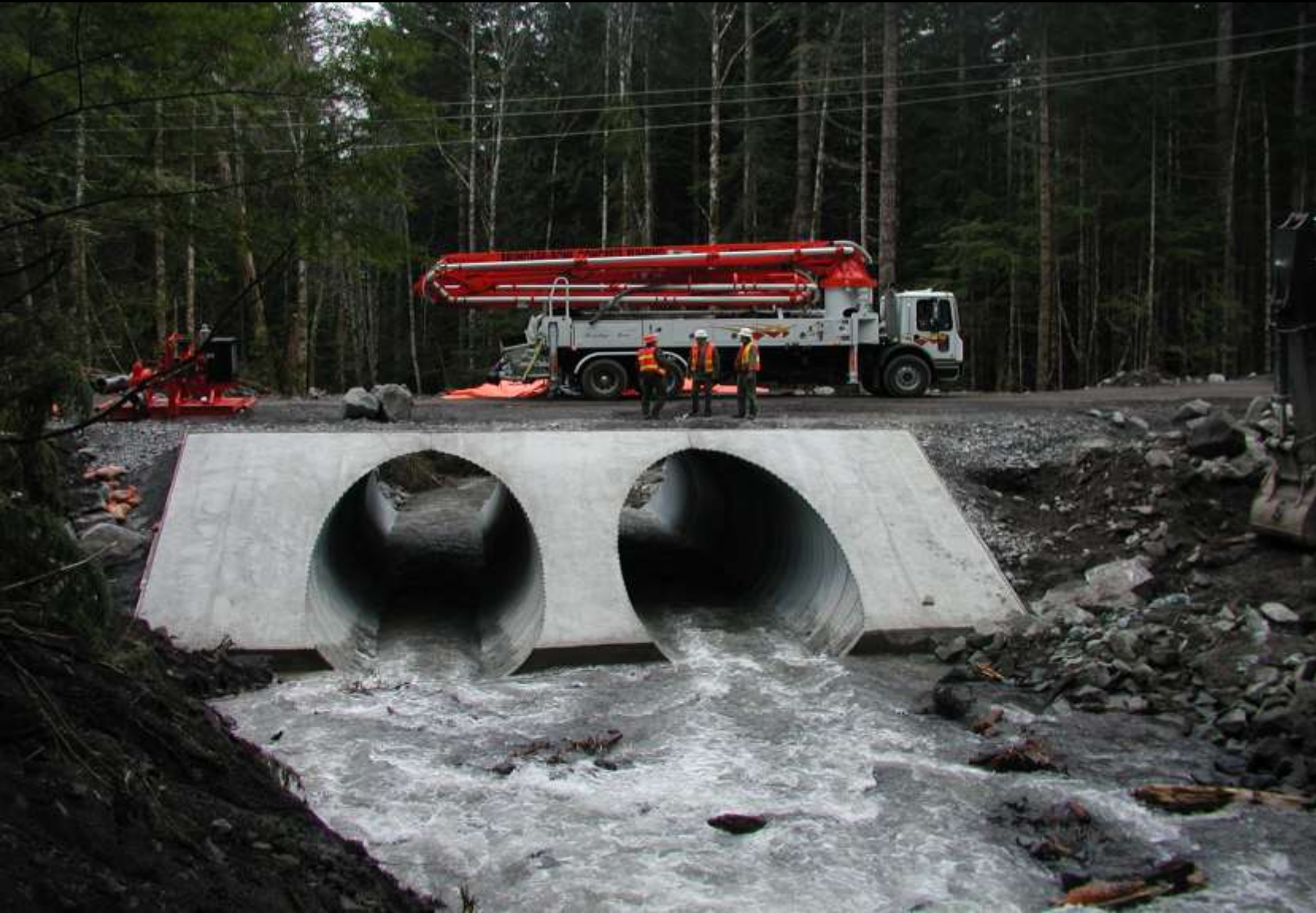
Kautz Creek culverts installation complete with water flowing on Friday April 27, 2007
