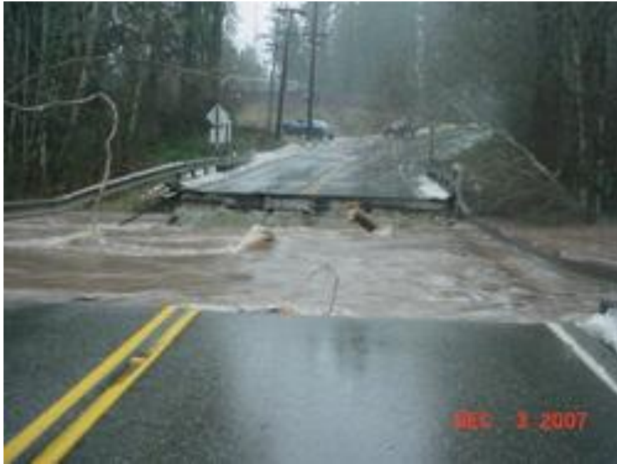
Dec 2007 Flood Damage Sauk River near Darrington
