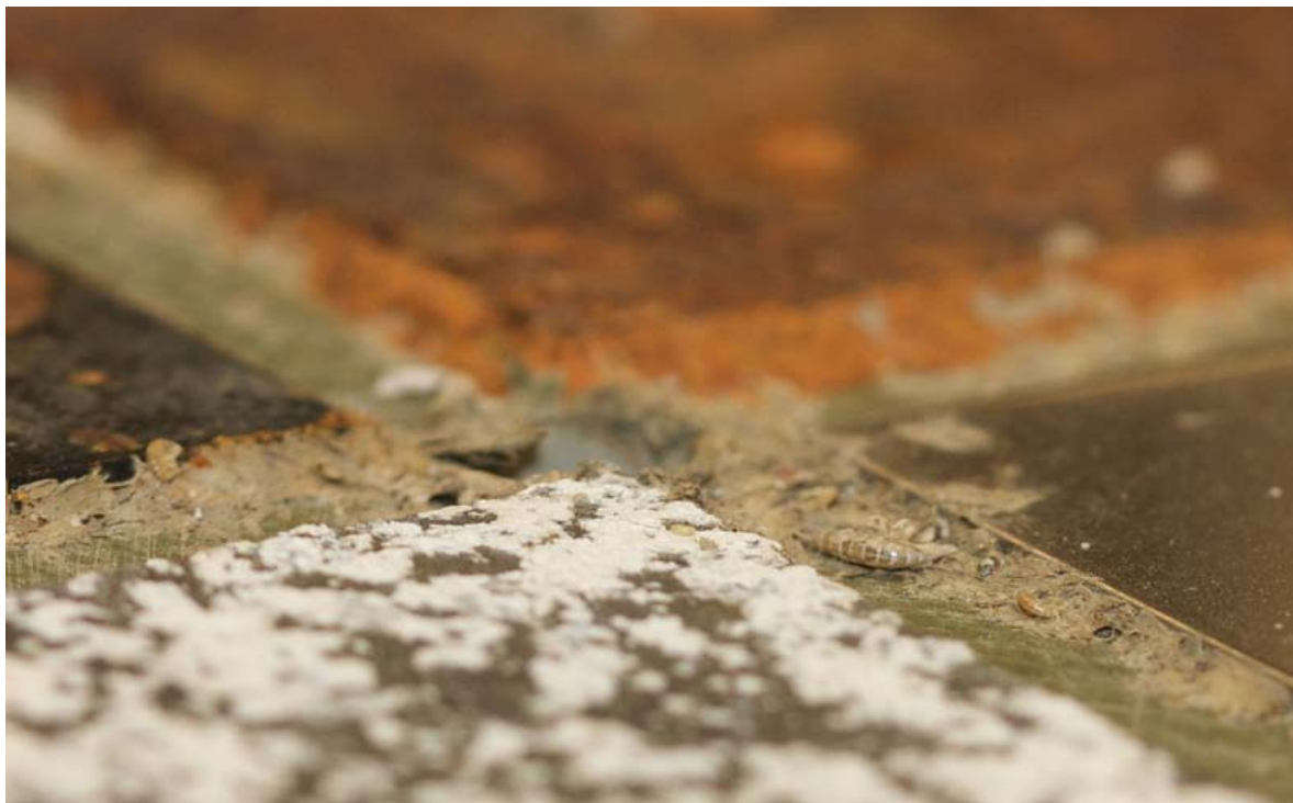
Figure 4.2 – Fouling and sediment deposition along edges and in crevices
