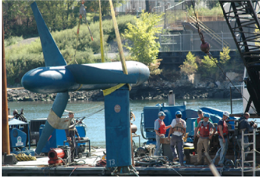
(a) Verdant tidal turbine
