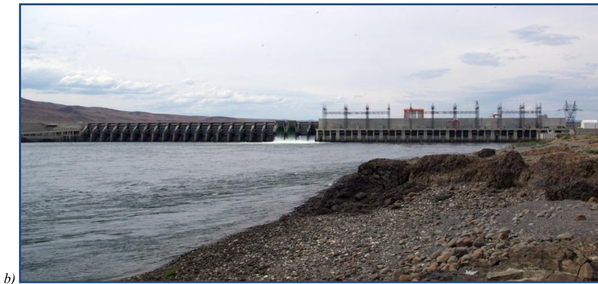
Figure 2.24 Images taken from the shore of the tailrace of a) the Wanapum Dam and b) the Priest Rapids Dam. Varying sized cobble stones are observed lining the banks. A ‘rib’ of exposed bed rock is seen in the bank of the Priest Rapids tailrace extending from near the center of the image to the right side of the picture.
