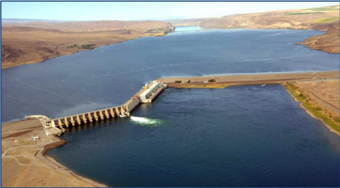
Figure 2.3 Aerial view of Wanapum Dam.
