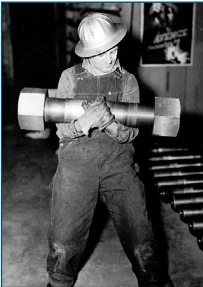
One-hundred, ninety-three pound nut and bolt, one of 16 used to join sections of the generator shaft of a 75,000 kW generator - Grand Coulee Dam, 1942
