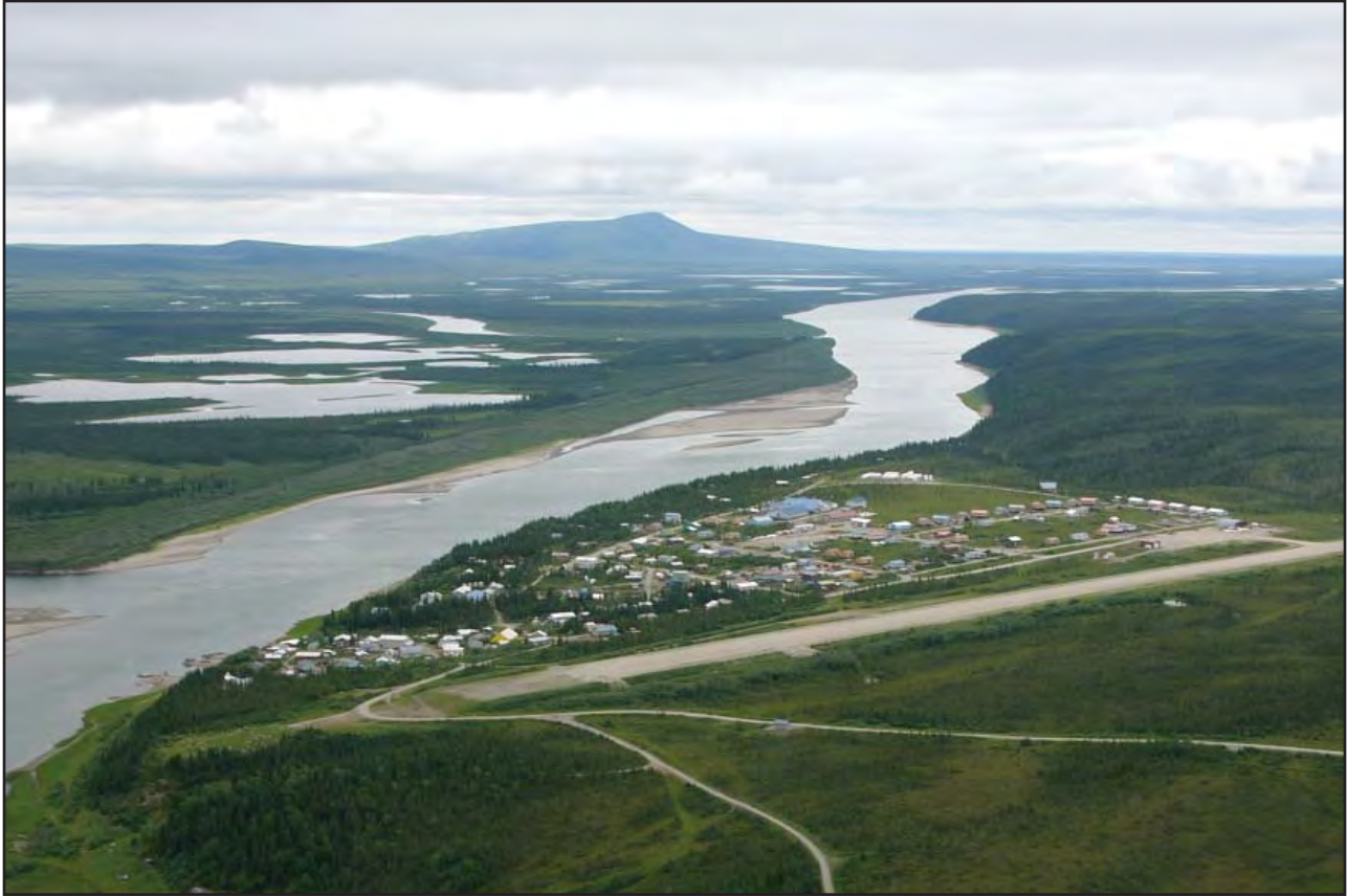
Figure 4-2.—Aerial view of Kiana, Alaska, looking southwest.
