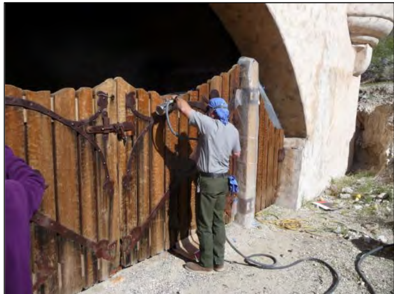
Applying consolidant with HVLP unit on 010E1GA03.
