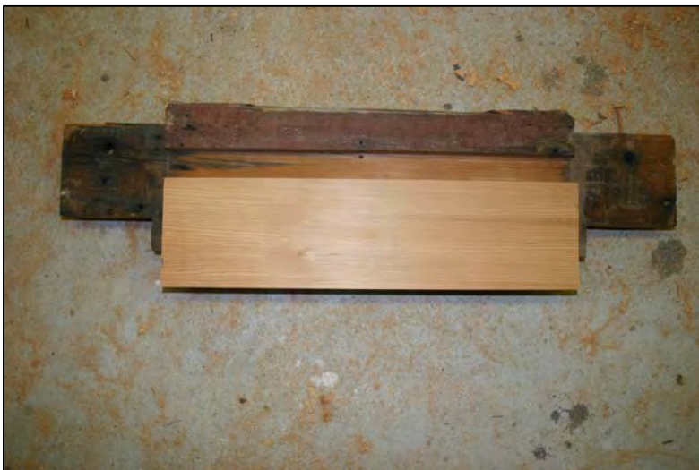
The bottom rail and dutchman insert prior to glue-up.
