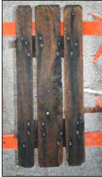
010E1SH003, wall face, after treatment
