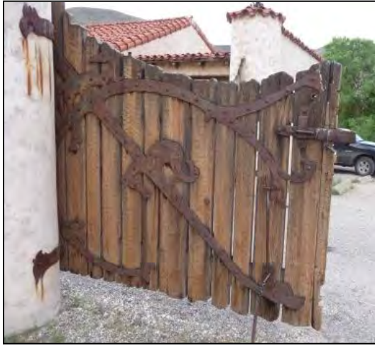
110W1GA001, west face before treatment
