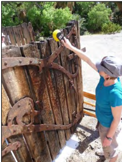
Acetone gel removal on west face of 010W1GA001.
