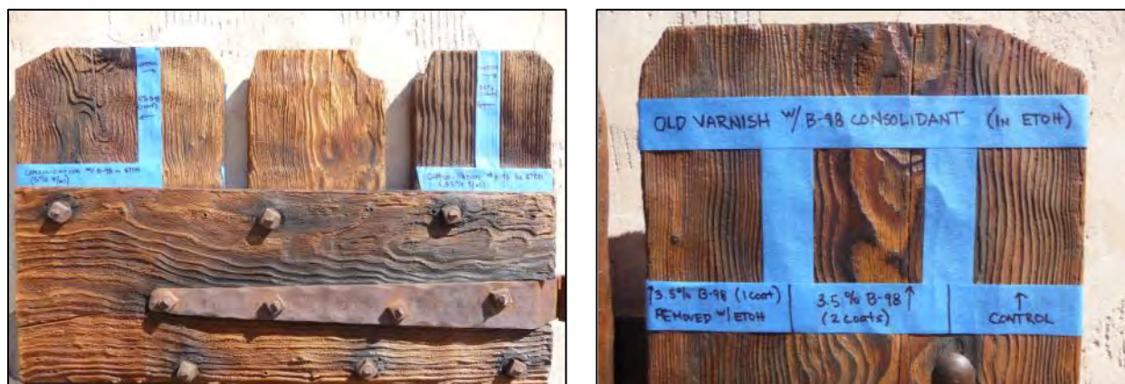
Test treatment areas on 010E1SH002
