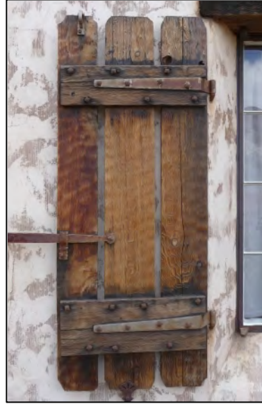
010N1SH001, exposed face, after treatment
