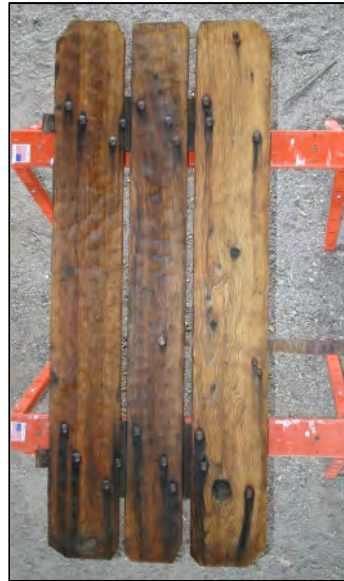
010E1SH001, wall face, after treatment
