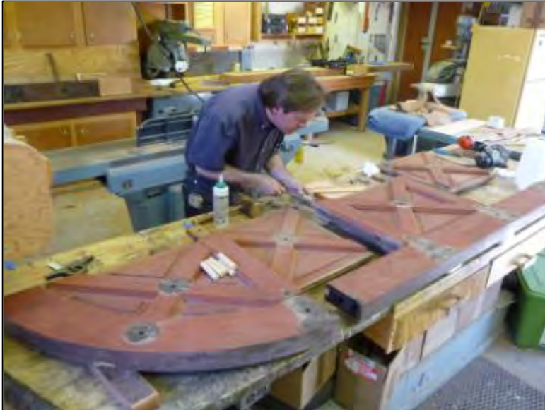
Disassembly of door at arch and lock rail.
