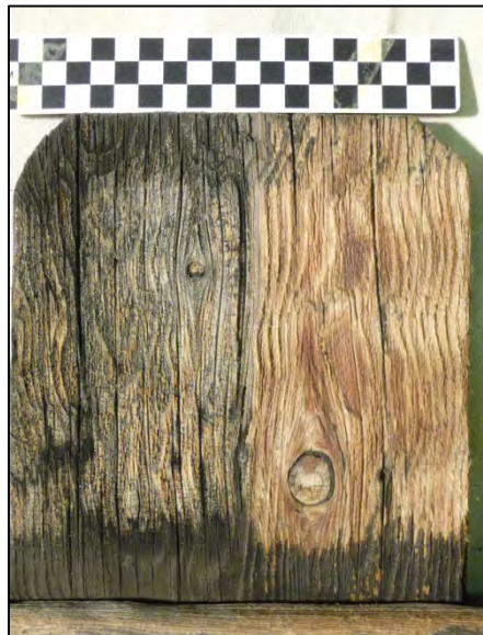
Mildew removal on exposed face of 010N1SH001
