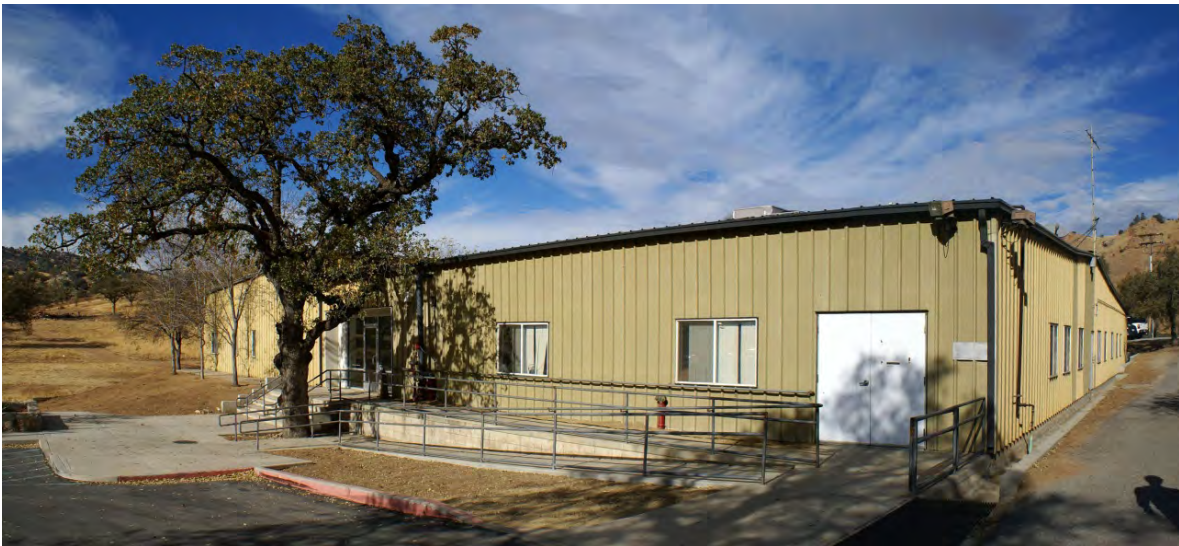
Buildings and Structures: The Administration building, looking northwest, shows the metal siding and the front entrance on the south side (PWR, CL Program, 2012).
