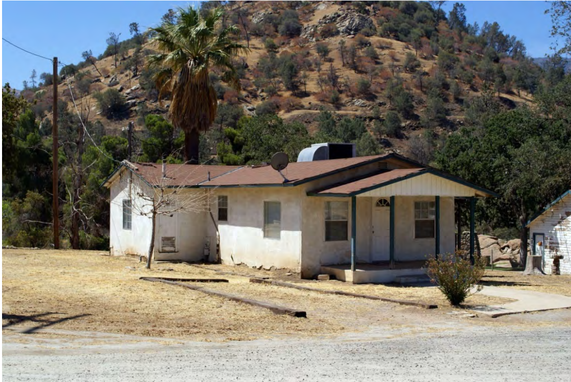
Buildings and Structures: Residence 9, looking southwest, shows the California bungalow influences, as well as the board-and-batten siding that was replaced with stucco in the 1950's (PWR, CL Program, 2014).
