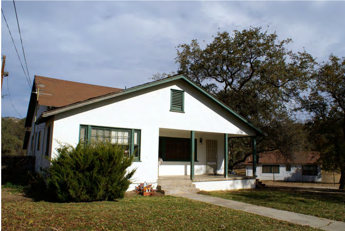
Buildings and Structures: Residence 13, looking east, was moved from its original location, near what is now the picnic area, to its present location in the 1950's (PWR, CL Program, 2012).
