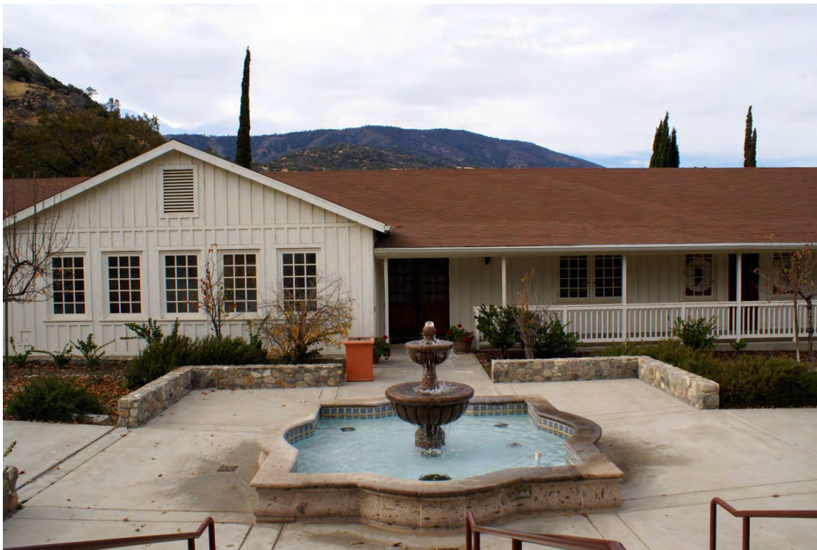
Buildings and Structures: The Visitor Center (building 2), looking west, was completed in 2004, but was built on top of the original building's 1914 foundation (PWR, CL Program, 2012).
