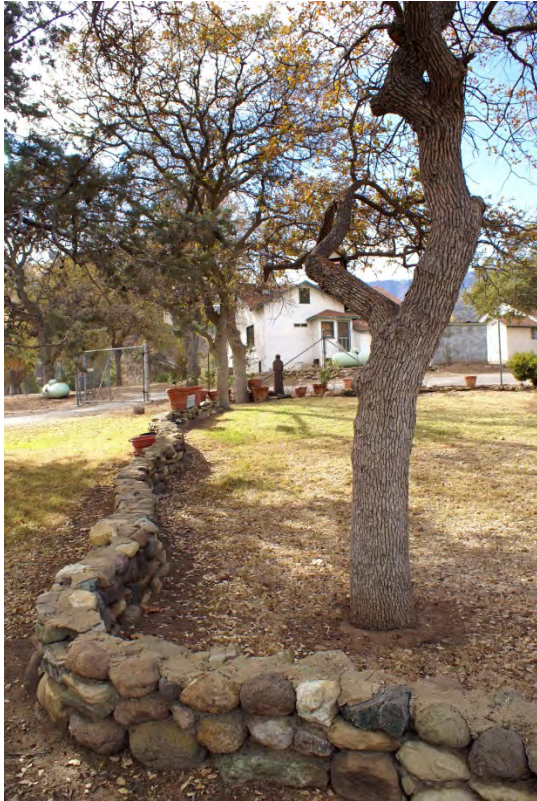
Small-Scale Feature: Looking west, the stone wall running the perimeter of the Chávez garden area is a combination of round river rock and concrete (PWR, CL Program, 2012).
