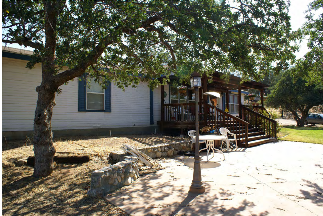
Buildings and Structures: House 20, looking east, is one of the last remaining structures within the manufactured housing area (PWR, CL Program, 2014).
