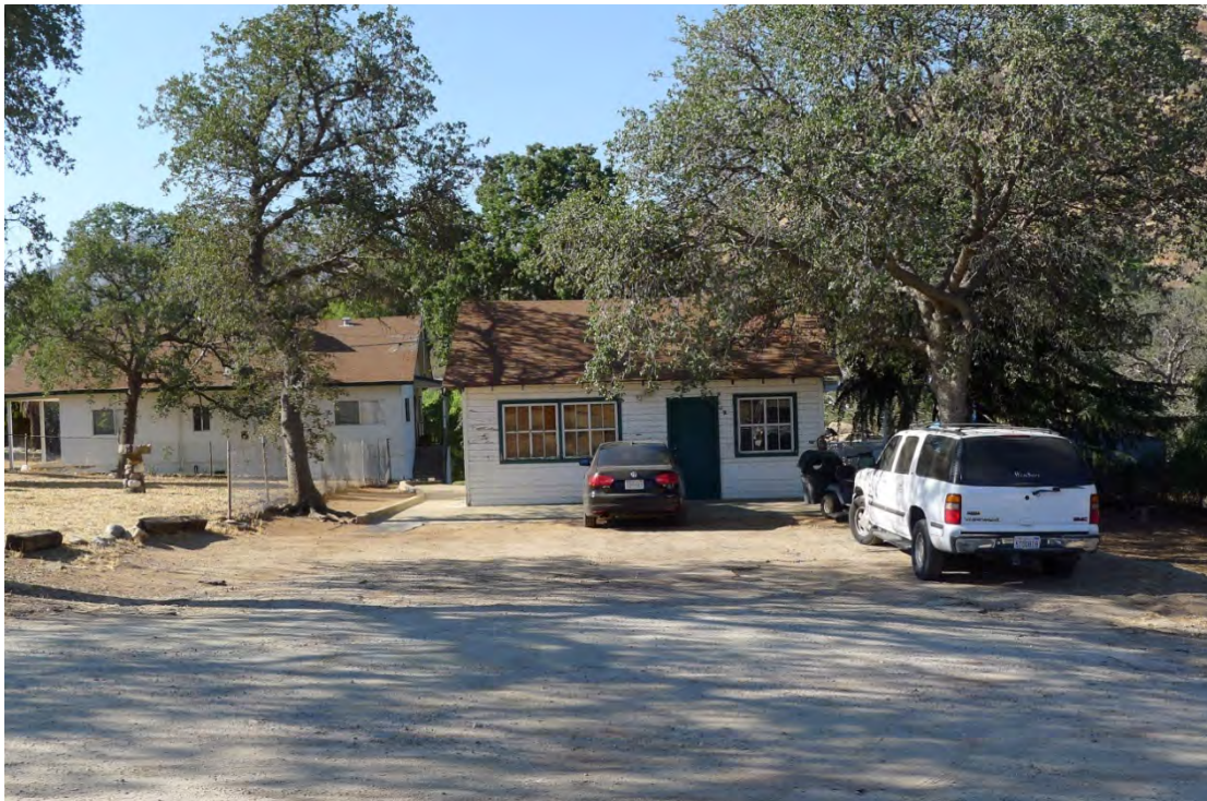
Buildings and Structures: Storage Unit Building 10, looking south, was built in the 1950's and shows its relationship with residence 9 in the background(PWR, CL Program, 2014).
