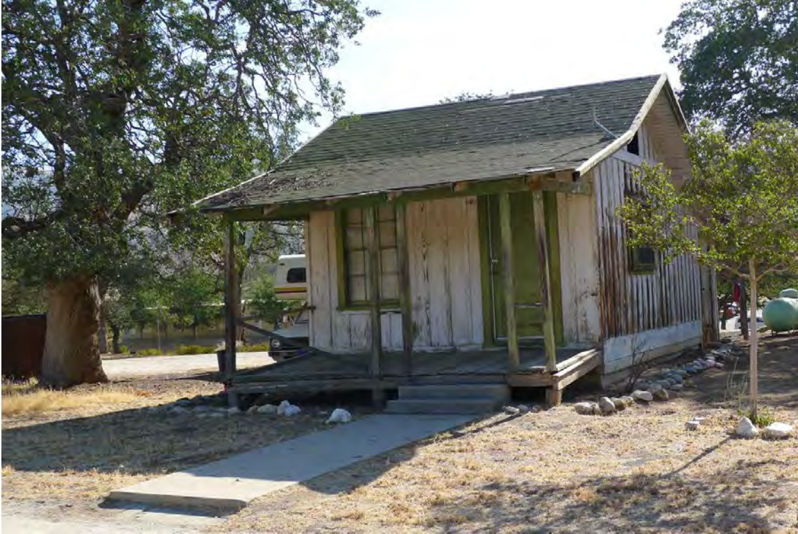
Buildings and Structures: Residence 11, looking east, shows the original board-and-batten siding (PWR, CL Program, 2014).
