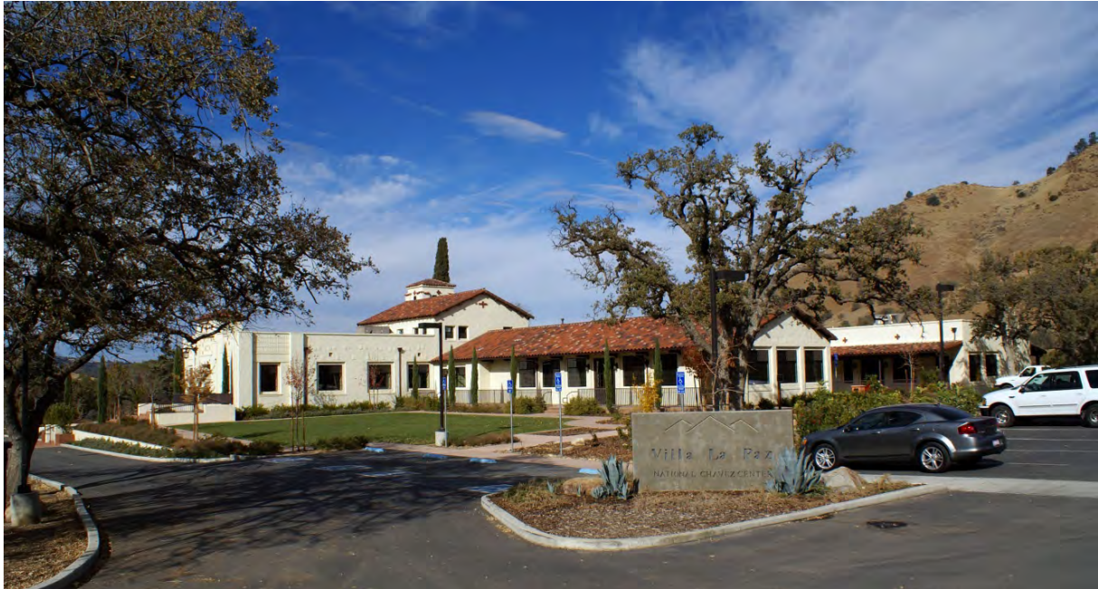
Buildings and Structures: The north unit, La Paz, is situated at the base of Three Peaks with its formal entry on the south end of the building (PWR, CL Program, 2012).
