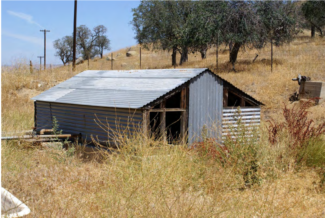
Buildings and Structures: The second settling ponds Pump House 2 (building 34), looking north, at the southern entrance of the pond area, north of Pump House 1 (PWR, CL Program, 2014).
