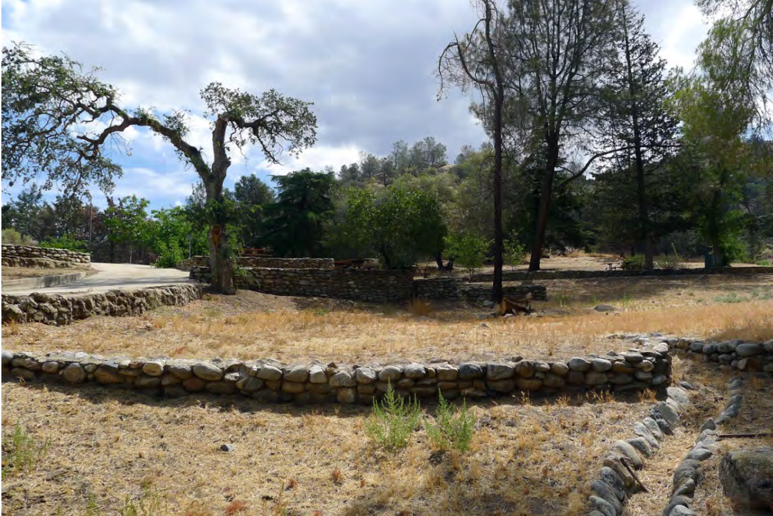
Small-Scale Features: The dry-stacked stone retaining walls define the picnic area just south of the Visitor Center (building 2) (PWR, CL Program, 2014).
