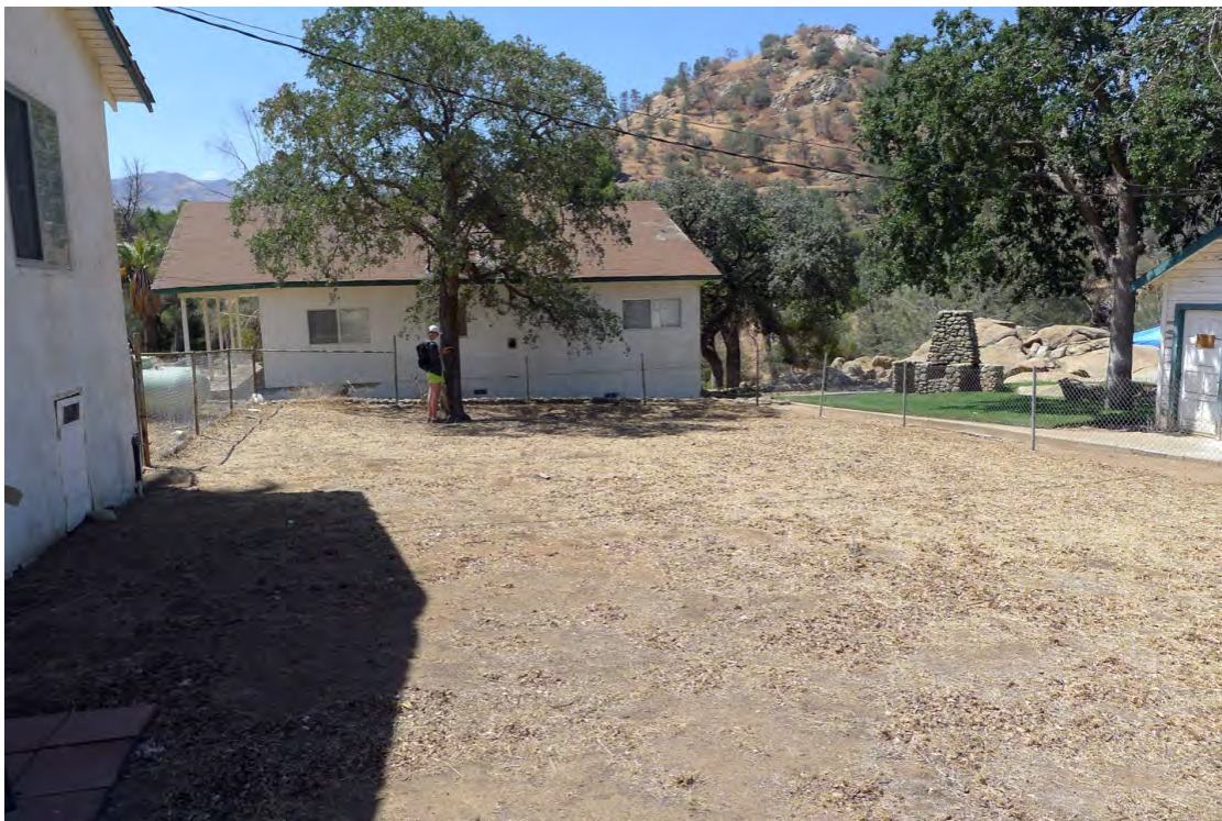
Small-Scale Features: Looking south, the chain-link fence that forms the backyard for residence number 9 can be seen in the background. The fence includes a metal gate on the east side (PWR, CL Program, 2014).
