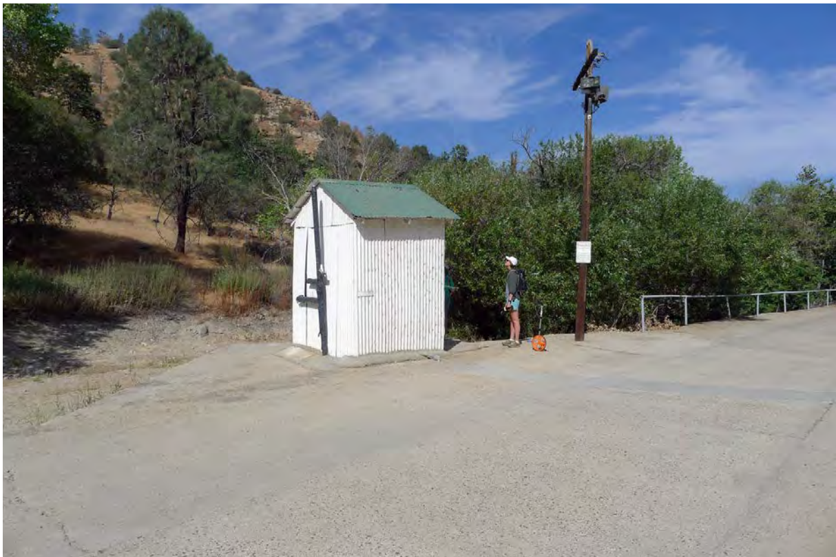
Buildings and Structures: The back side of the South Pump House (building 31), looking northwest, showing the location in relation to Tehachapi Creek (PWR, CL Program, 2014).
