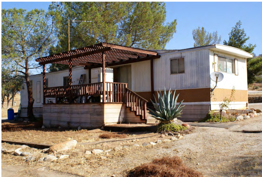
Buildings and Structures: This manufactured house (building 21), looking northeast, is the last remaining single-wide trailer of twenty that once resided in the manufactured housing area (PWR, CL Program, 2014).
