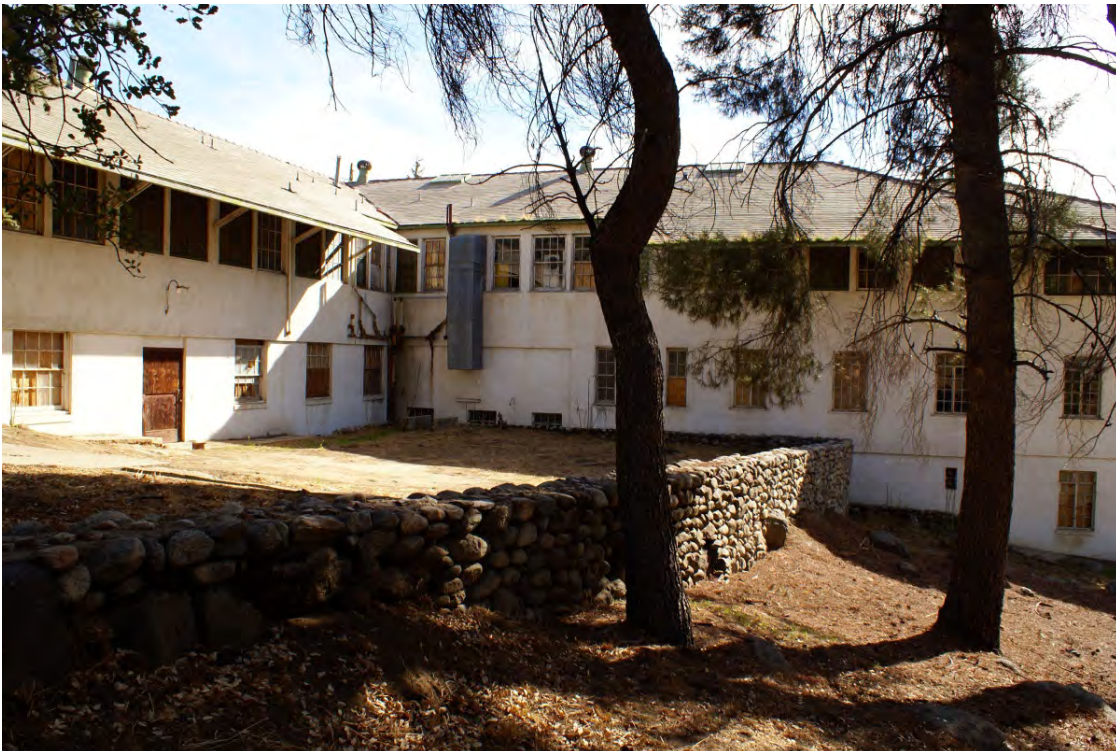
Small-Scale Feature: This stone retaining wall, looking south, is located on the north side of the Dormitory (building 4) building, and provides a leveled area at the terminus of the adjacent paved driveway (PWR, CL Program, 2012).
