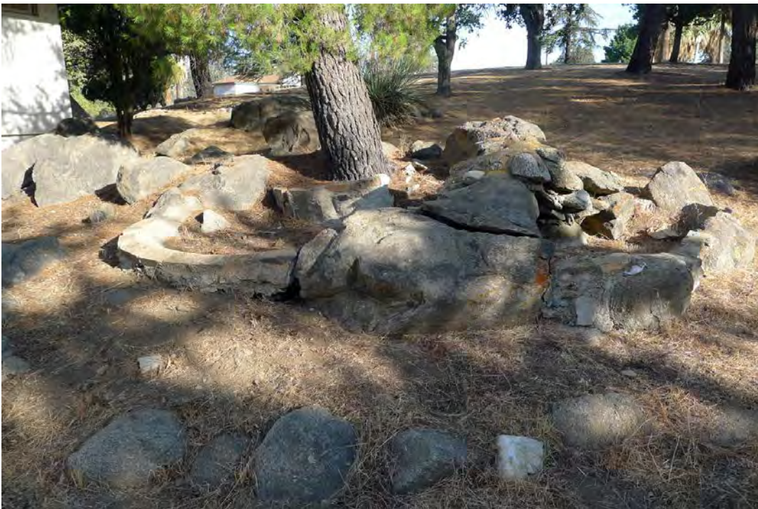
Constructed Water Features: Looking north, what remains of the fish ponds includes three tiers of stone and concrete walls and metal water pipes (PWR, CL Program, 2014).
