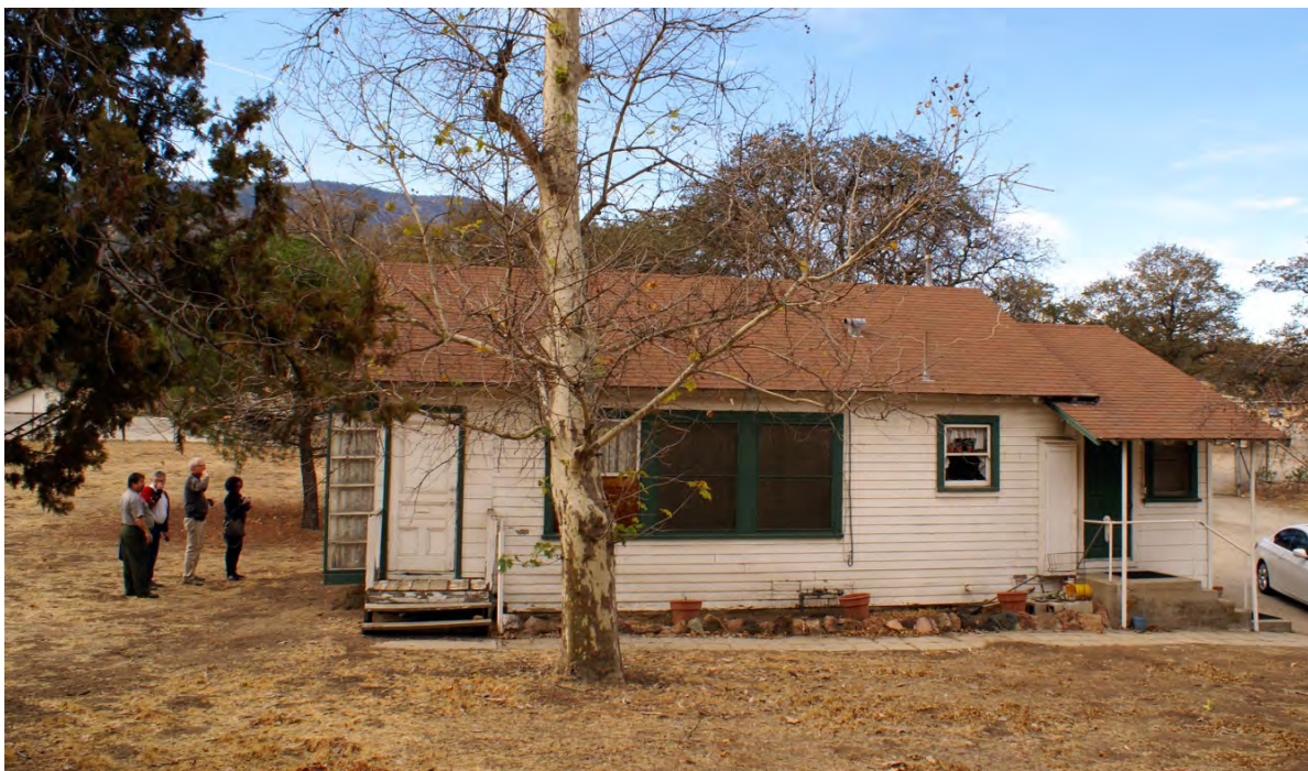
Buildings and Structures: The Chávez house, looking west, is a single story structure that was home to the Chávez family and where Helen Chávez still resides (PWR, CL Program, 2012).
