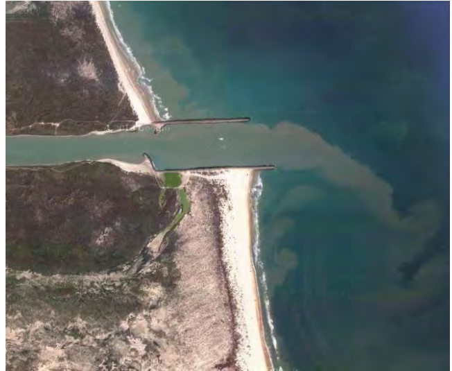
Photo 30. Imagery of Mansfield Channel jetties at the southern boundary of PAIS shows the flow of sediments through the channel and away from the littoral nearshore zone (Source: Google maps imagery https://maps.google.com , 2013).
