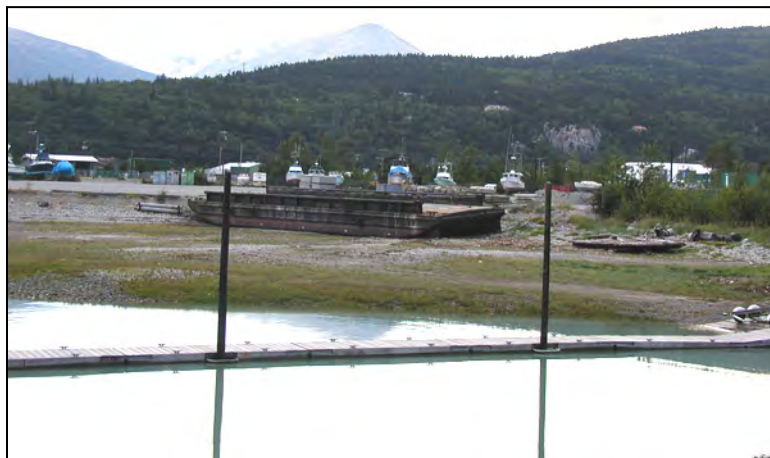
Figure 2-7. Beached barge on the north side of the Small Boat Harbor, Skagway. This beach could be at the same approximate elevation as the Gold-Rush era beach elevation at low tide. The barge is important for its association with the lighters and barges of the era of historical significance (although the barge itself is not historic) (July 2004).
