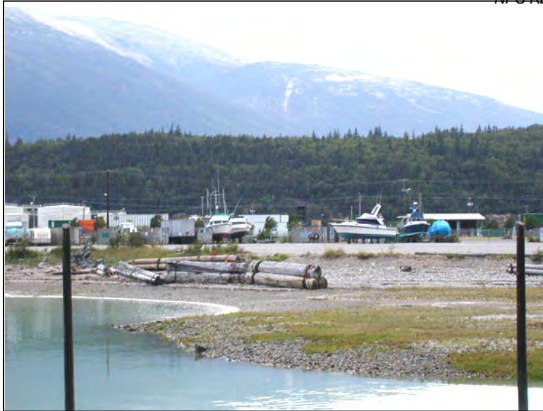
Figure 2-6. Old pilings discarded on the beach. West side of the Small Boat Harbor. It is not clear in which era these pilings were built, but they represent, in general, the methods of wharf construction that date back to Skagway's early years (July 2004).
