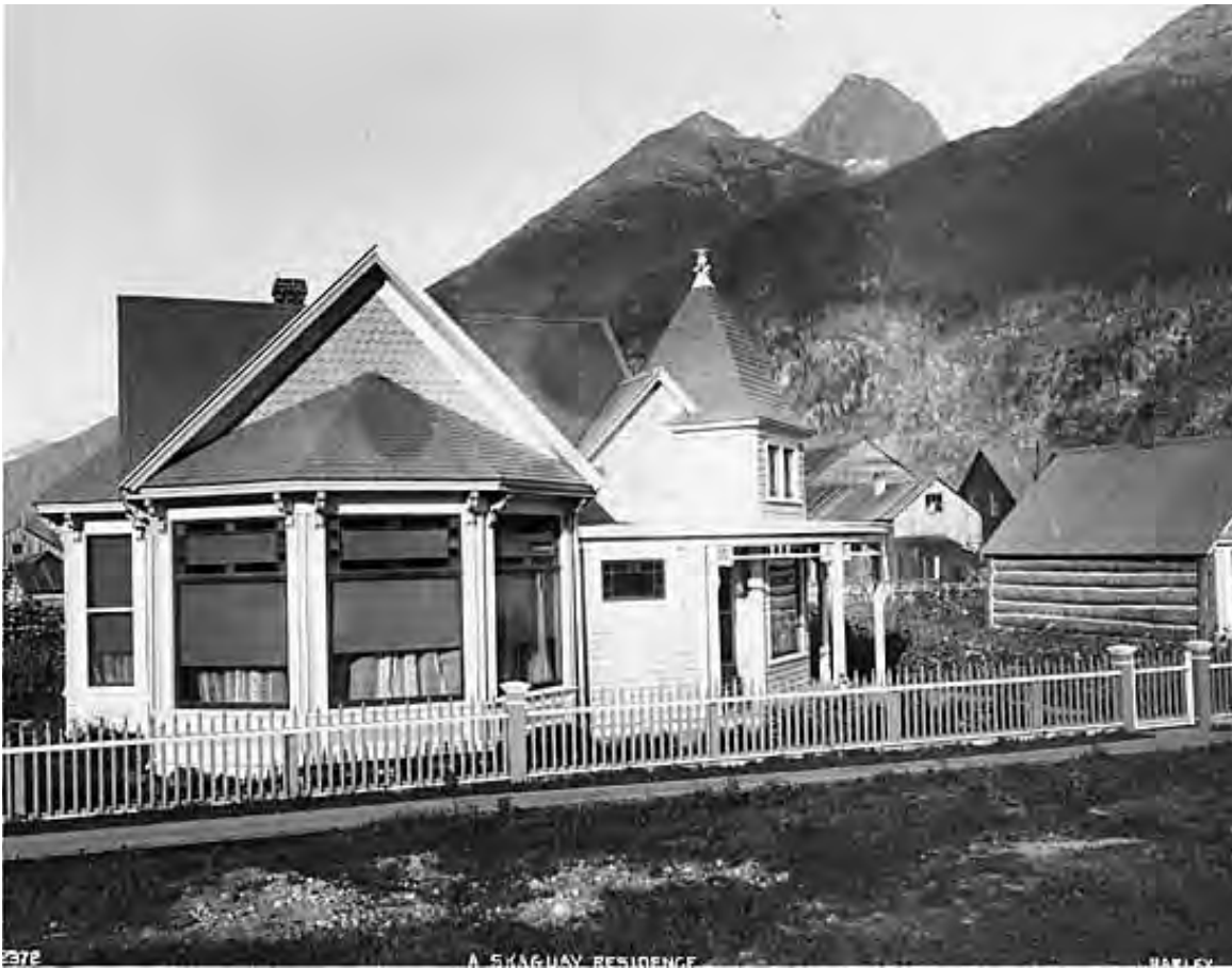
Figure C.11 A Skagway residence. [Exterior view of a frame home of a rather composite structure (it appears as though three cabins have been joined together). It also features a rounded porch and small cupola on top.] Date: [1902] Fonds/Collection: H.C. Barley fonds Photographer: H.C. Barley Yukon Archives PHO 5054
