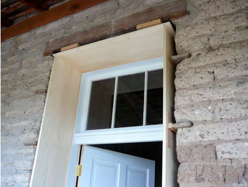
Figure 3. Several remaining door casings were completed, including this one on the north wall of the Surgeon's office in the Administration Building.
