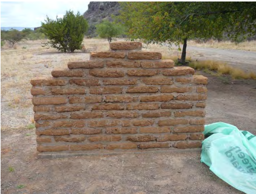
Figure 4. Construction of an adobe test wall.
