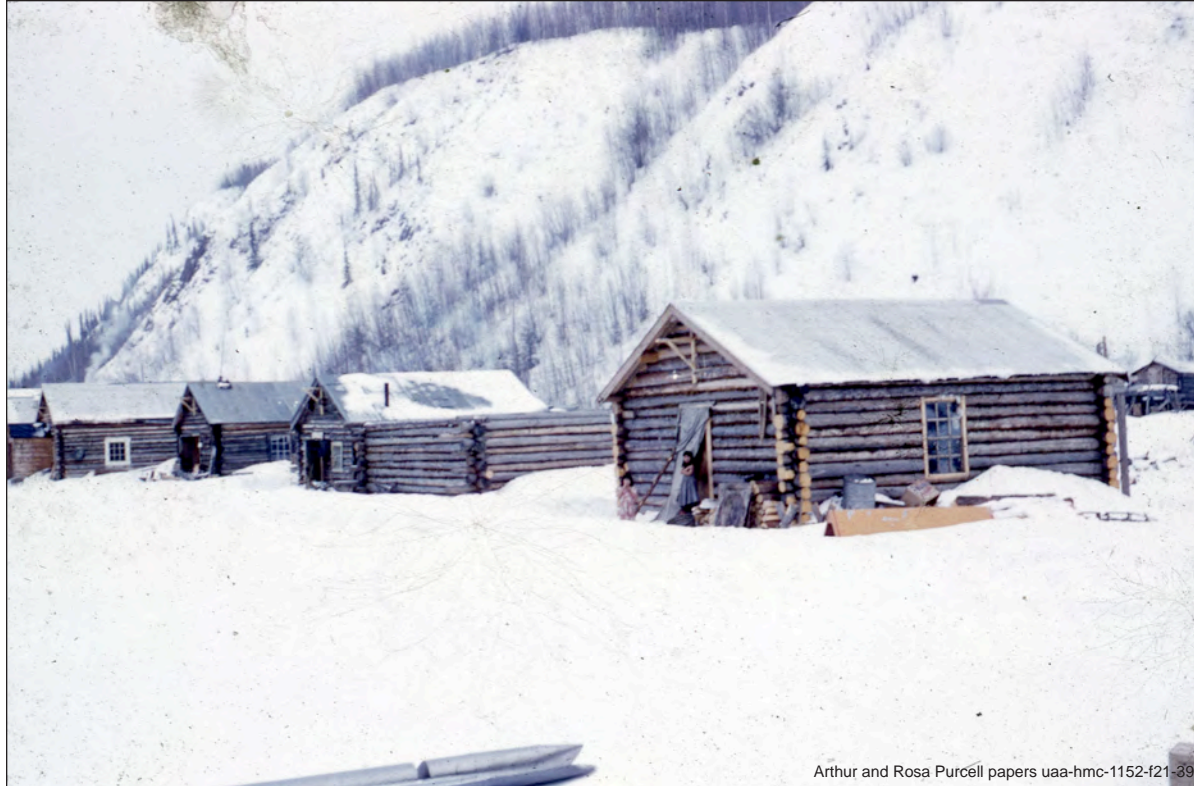
Plate 3-1.—A view of the northern section of housing in 1957.
