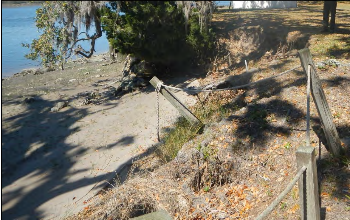
Figure 15. “End-around” erosion south of a stabilized shoreline area at Plum Orchard (SMUMN GSS photo).
