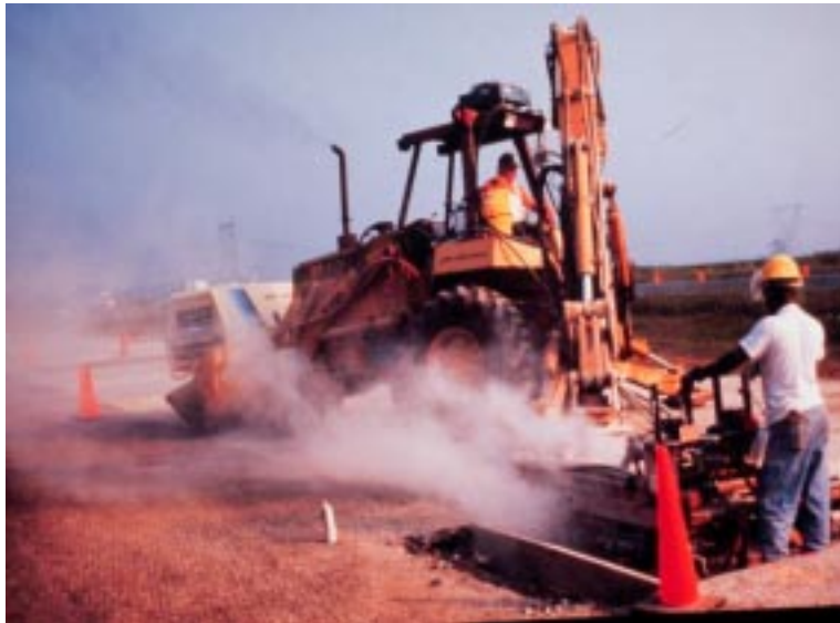
Construction worker exposure to silica dust while drilling concrete pavement during interstate highway repair.
