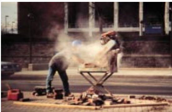
Silica dust exposure to construction worker sawing masonry brick without dust control or a respirator.
