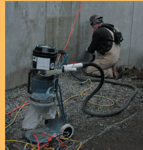
Vacuum and shroud on grinder
