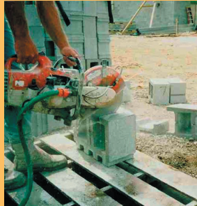
Water spray from hose
