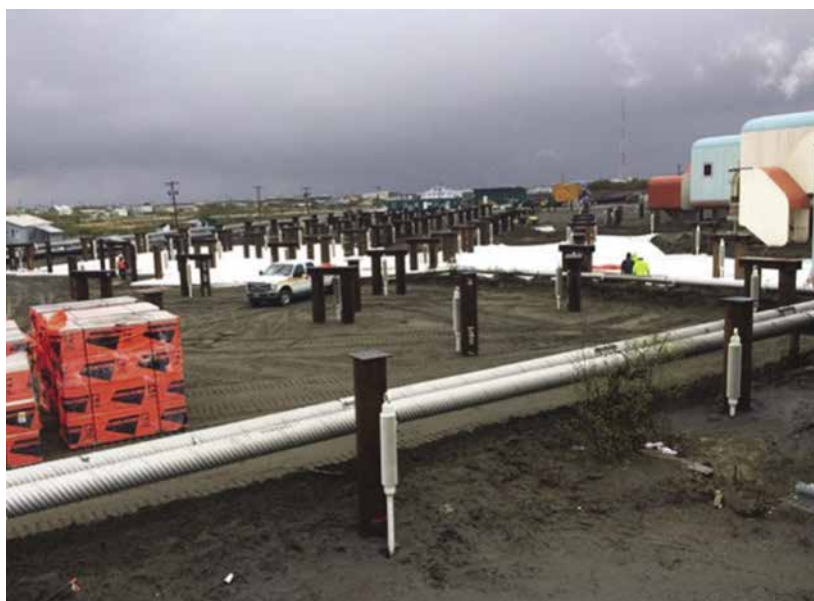
Figure 3-6. Driven pile foundation with thermosyphons for new hospital and clinic expansion.
