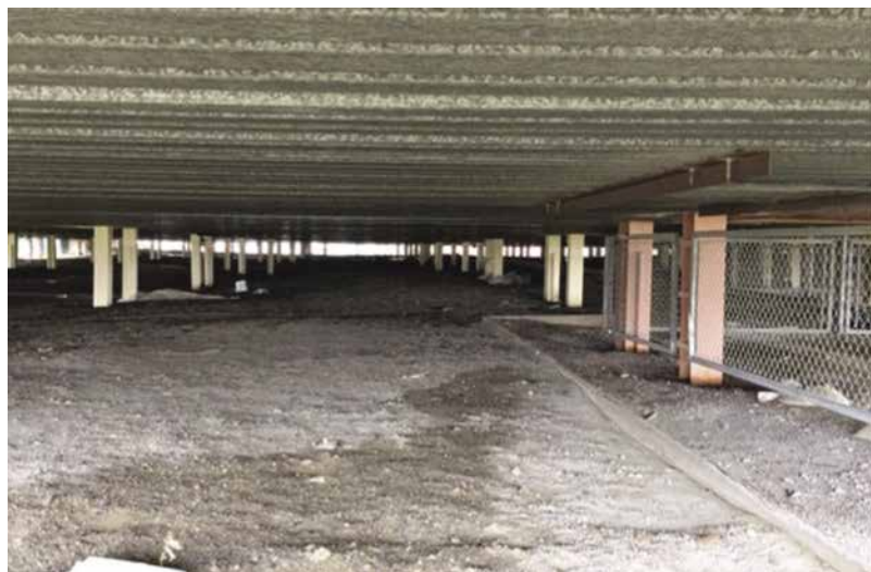
Figure 3-5. Driven pile foundation supporting the existing clinic. Square tubes attached to the piles may be used for temperature monitoring and passive or active cooling of the surrounding permafrost.
