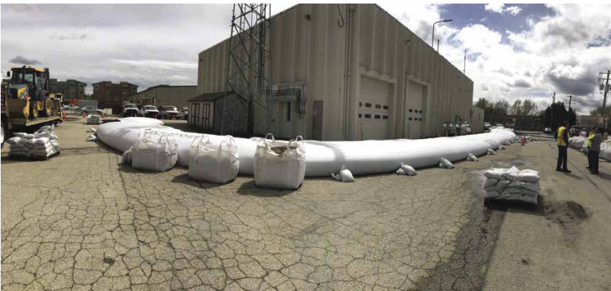
Figure D-3. Installed water-filled cofferdam.
