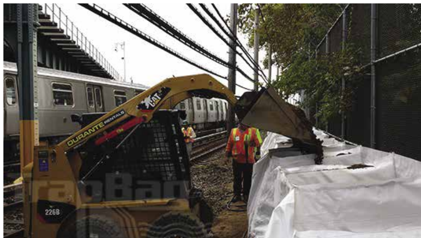
Figure D-11. Installation of TrapBag system.
