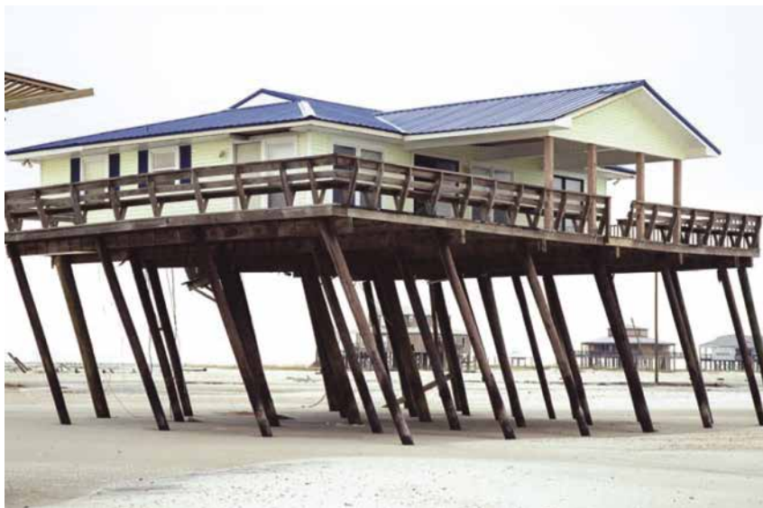
Figure 7-19(a). Structure near collapse because of insufficient pile embedment before Hurricane Katrina, Dauphin Island, AL. Source: FEMA (2009).
