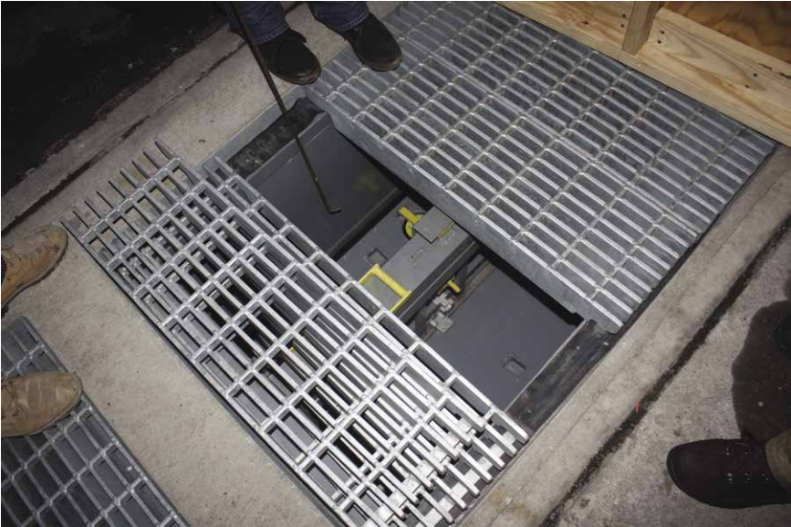
Figure D-7. Installation of mechanical closure device. Source: Courtesy of FloodBreak (reproduced with permission).
