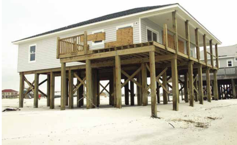
Figure 7-19(b). The same structure as that shown in Figure 7.19(a) after Hurricane Katrina, Dauphin Island, AL, with a successful pile foundation that supported the elevated home even after scour and erosion removed several feet of soil. Source: FEMA (2009).
