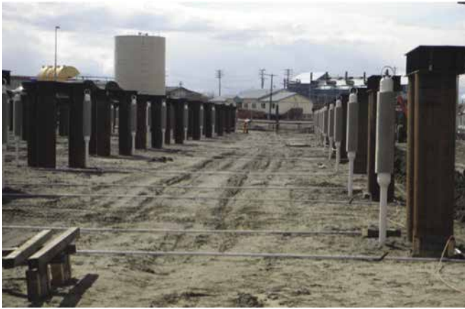
Figure 3-7. Flat-loop evaporator system installed during construction (white PVC pipes). The system will be used if permafrost temperatures rise to levels greater than anticipated under the most-probable condition.
