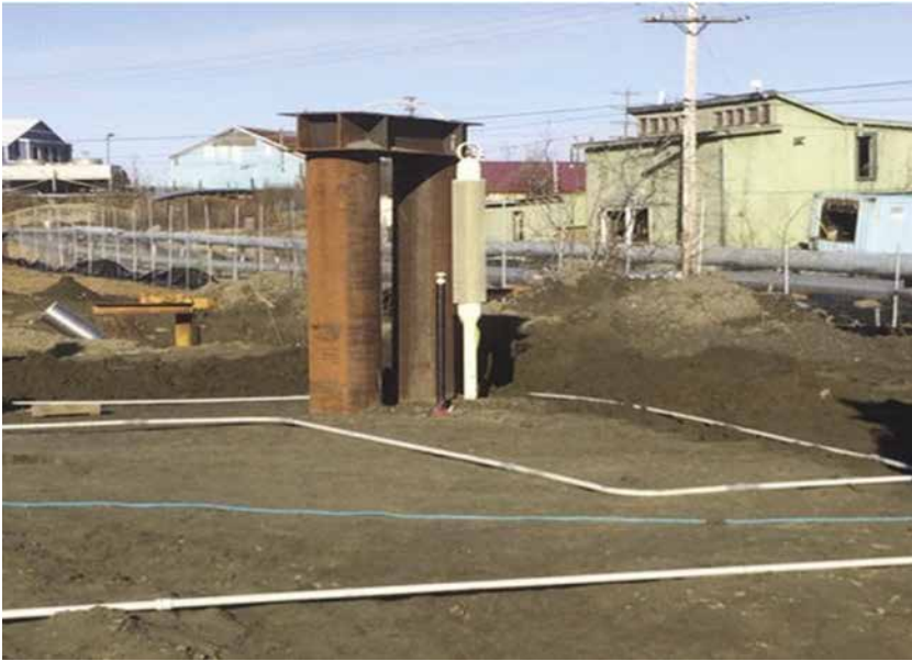
Figure 3-8. Temperature-monitoring well (black plastic pipe) adjacent to driven pile and thermosyphon.
