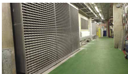
Figure D-9. Typical louvered vent panel.
