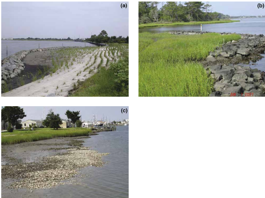
Figure 7-25. Shoreline stabilization projects in North Carolina illustrating the living shoreline approach. (a) Project to replace failing seawall included fill, marsh transplants, and rock sill; here shown 2 years post-construction. (b) Project to protect the marsh edge, which included rock sill, no fill, and minimal transplants; here shown 4 years post-construction. A drop-down in the sill provides marsh access to nekton. Oysters can be seen colonizing the lower rock surfaces. (c) Project to protect eroding sandy beach includes only natural habitats, achieved with salt marsh transplants and oyster reef restoration; shown here 4 years post-installation.
