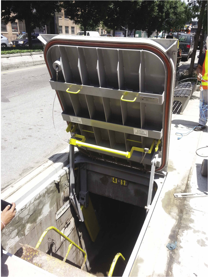
Figure D-22. Watertight emergency egress hatch. Source: Courtesy of Walz & Krenzer (reproduced with permission).
