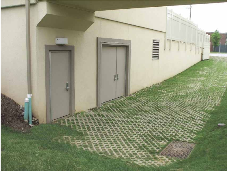
Figure D-27. Fire-rated watertight doors installed.
