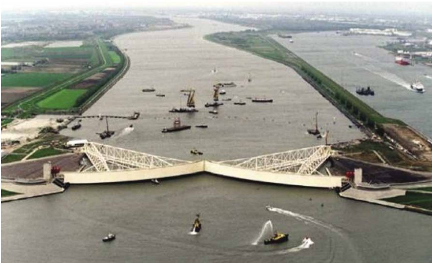
Figure 7-23. Maeslantkering, Nieuwe Waterweg, closed. Source: World66 (2011).
