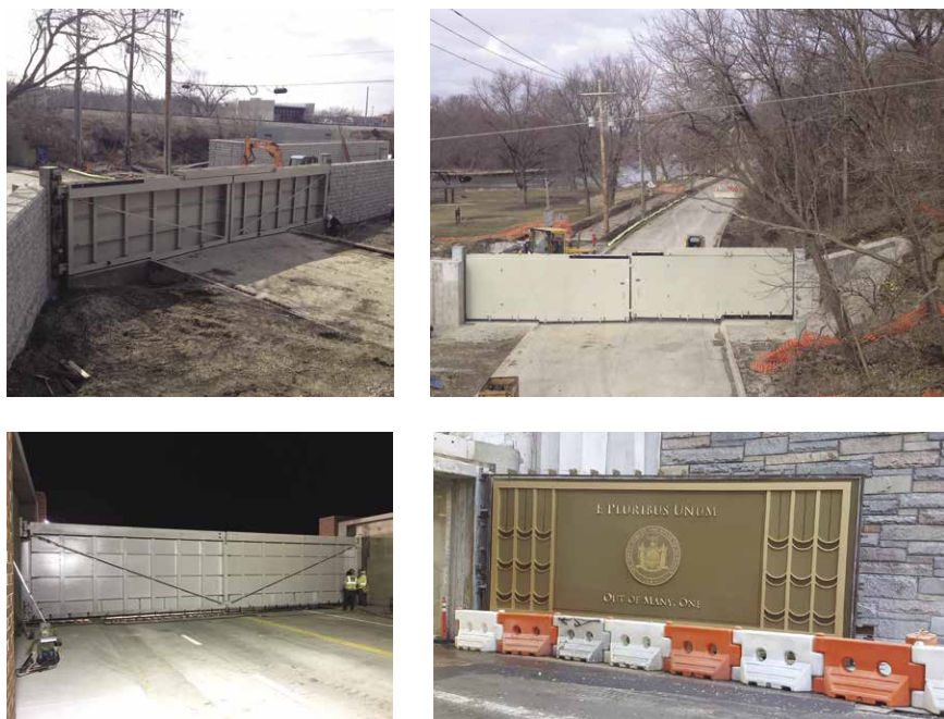
Figure D-20. Hinged watertight flood gate installations.
