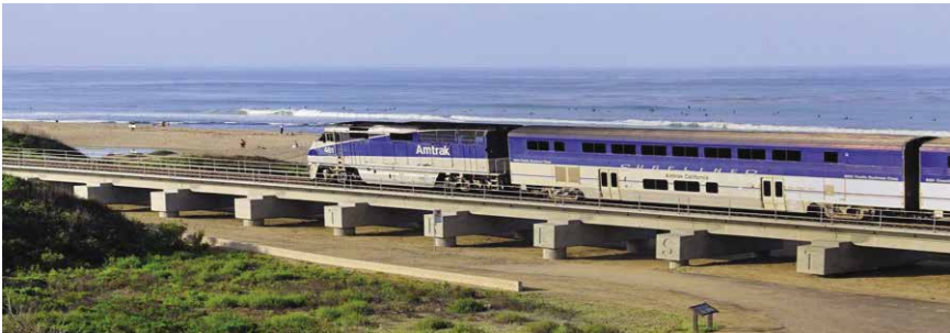
Figure 3-3(a). Los Angeles to San Diego (LOSSAN) Rail Corridor that follows the sea coast and crosses low-lying areas on trestles. Source: Dial et al. (2014).
