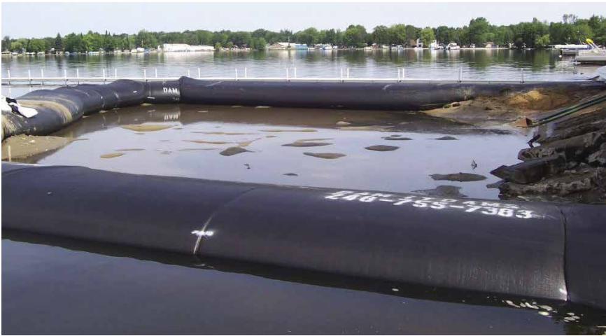
Figure D-2. Installed water-filled cofferdam.
