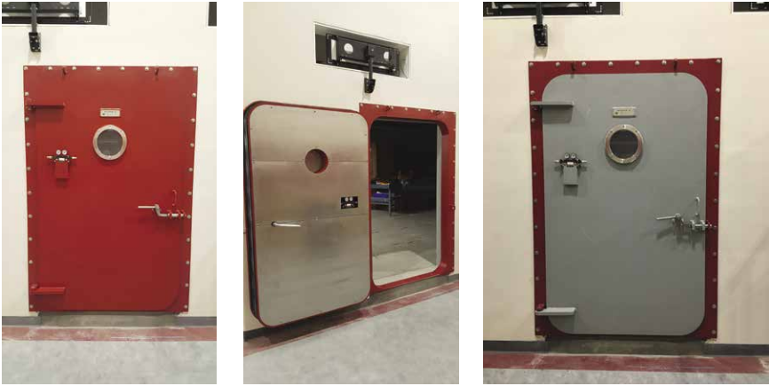
Figure D-21. Hinged watertight marine doors installed.
