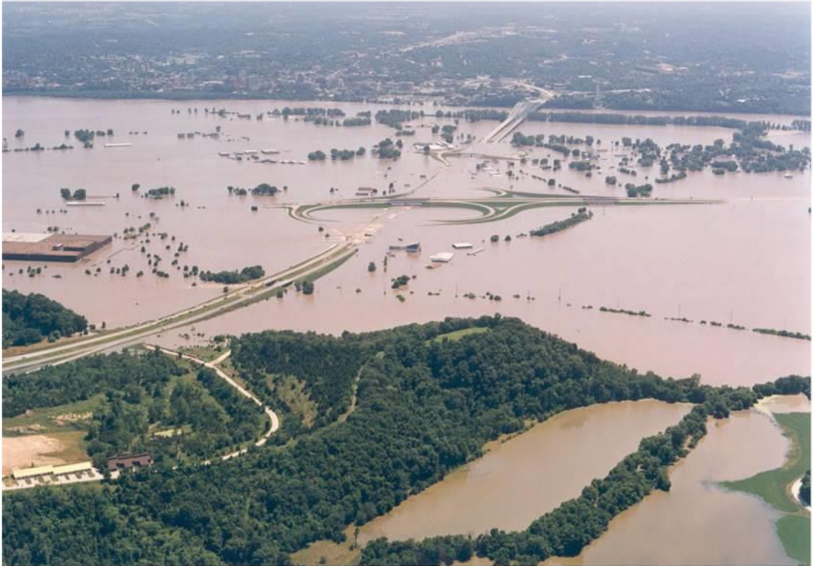
Aerial view of the Missouri River flooding on July 30, 1993, in the vicinity of Cedar City and Jefferson City Memorial Airport immediately north of Jefferson City, Missouri, looking south (photograph from the Missouri Highway and Transportation Department).
