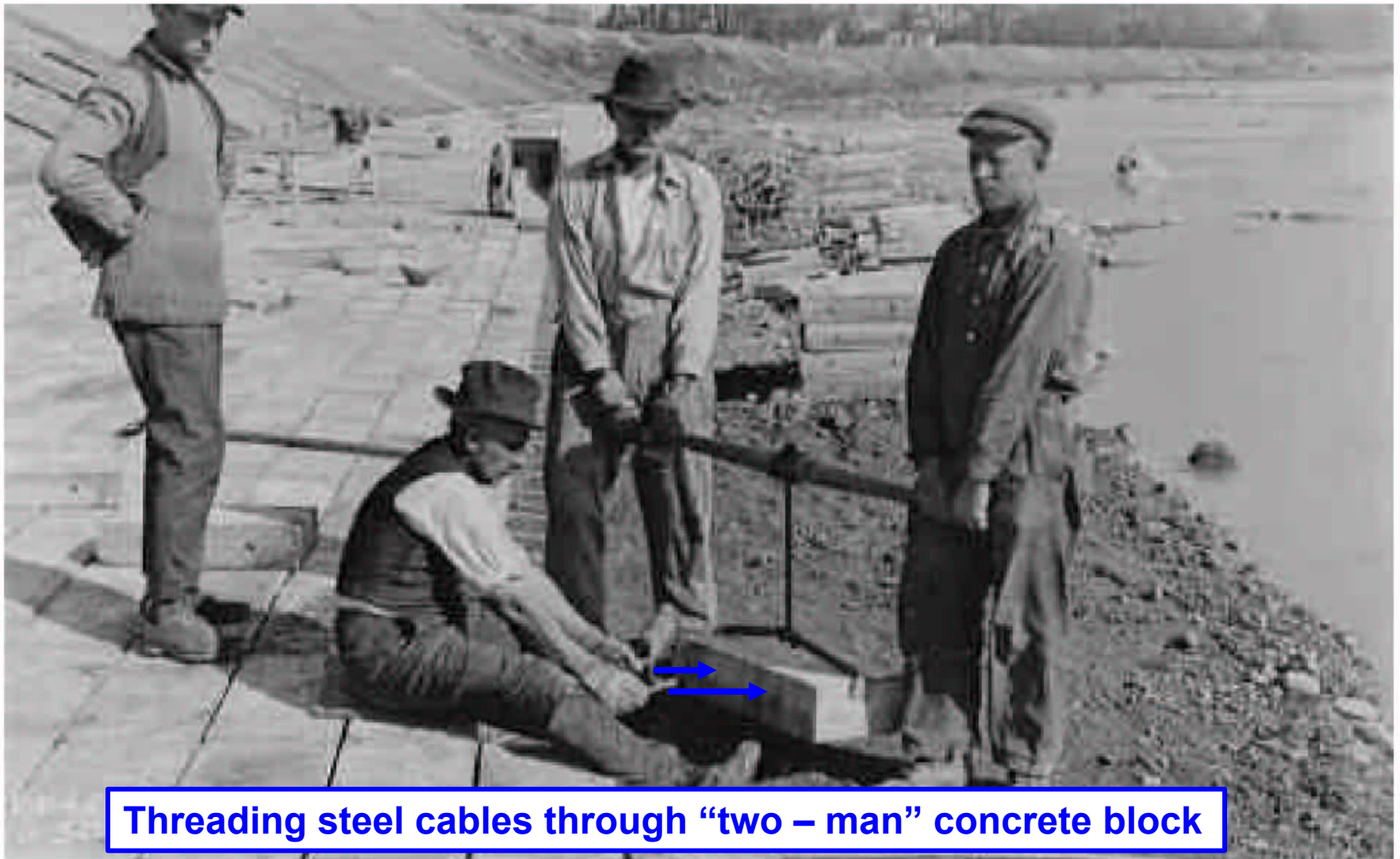
Figure 71 Dayton Feature - Laying blocks for flexible revetment . Looking upstream of Great Miami River. McKinley Park sewer outlet in slope
