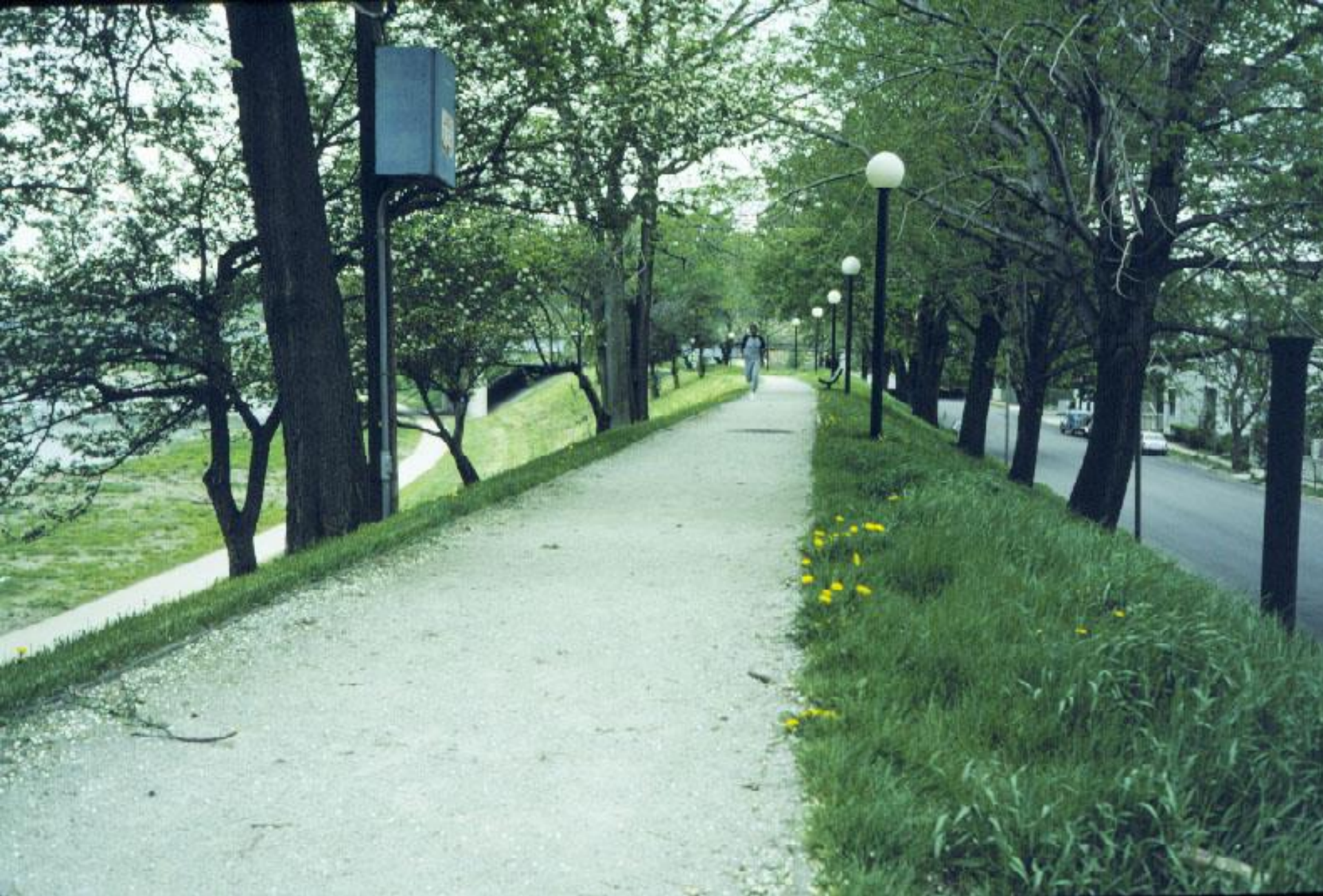
Great Miami River near Dayton - Levee section – Recreation paths
