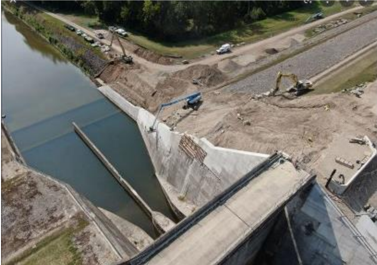
Example - Lockington Dam Concrete replacement 2020 - Sunesis Construction
