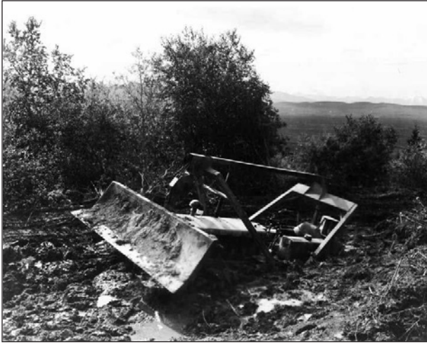
FIGURE 2 Permafrost-related challenges experienced during construction of the Alaska Highway, circa 1942. Surficial disturbances such as removal of overlying vegetation can cause rapid near-surface permafrost thaw, resulting in decreased bearing capacity of the soils. While the mired bulldozer shown here likely represented a mere inconvenience to the construction crew, permafrost thaw under permanent structures such as roads, pipelines, and buildings can cause major structural damage. Photo credit: Alaska State Library, Alaska Highway Construction Photograph Collection, ASL-P193-023.
