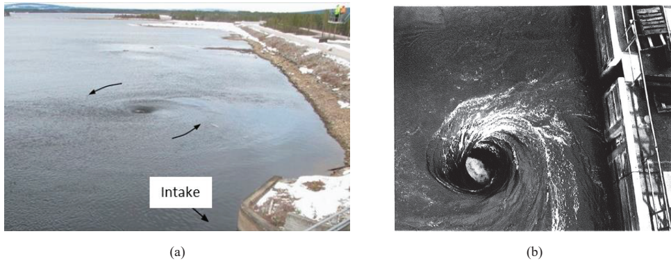
Figure 6.1 | Views of vortices at dam intakes: (a) occurrence of an intake vortex in a reservoir (Yang et al., 2018); and (b) vortex formation due to flow separation around the leading edge of a pier at an intake (Rindels and Gulliver, 1983).
