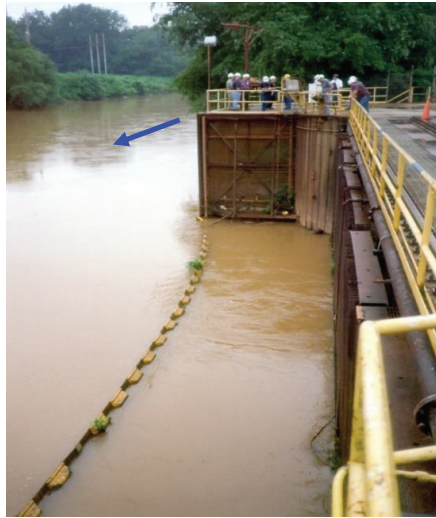
Figure 7.2 | A large, pump intake adjoining a bank of the Chattahoochee River, Georgia. The arrow indicates flow direction in the river.
