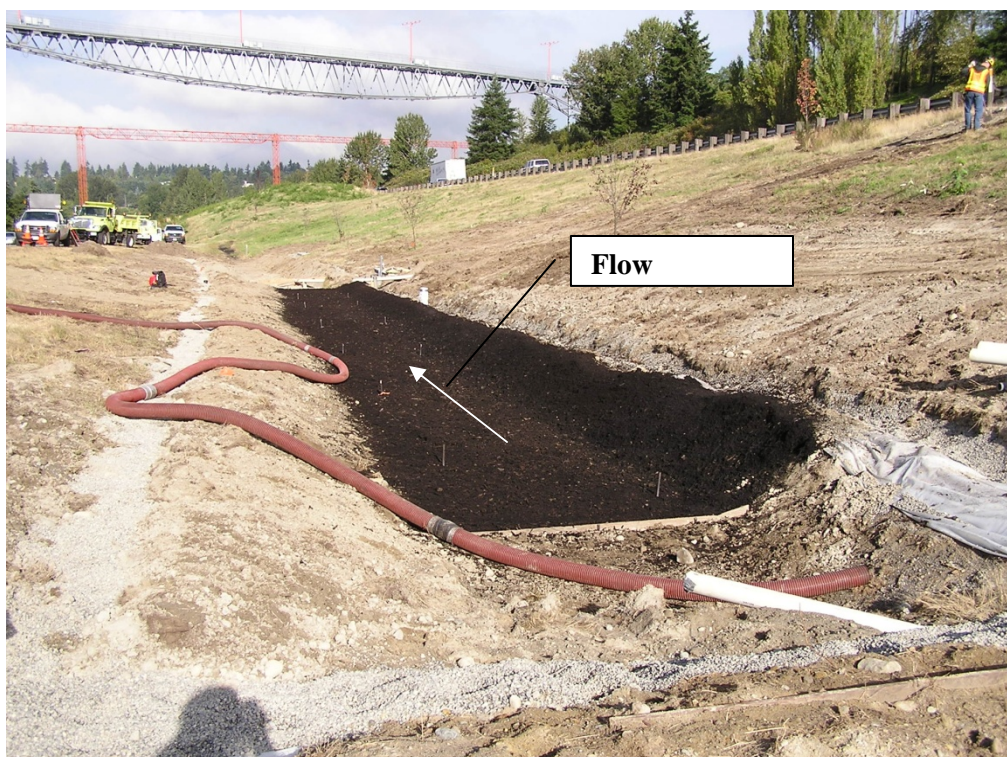
Figure 29. Bioswale with compost blanket installed
