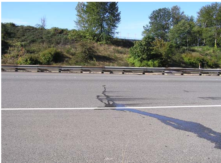
Figure 8. Water flow across the travel lanes from north to south towards curb
