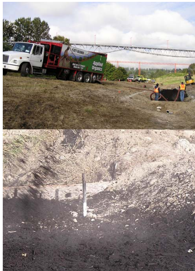
Figure 18. Compost blower truck (top) and steel pin showing final compost depth
