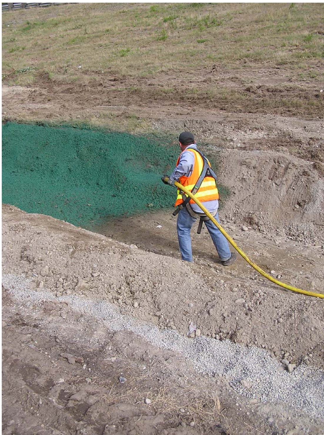
Figure 31. Hydroseeding Bioswale 2 with hose
