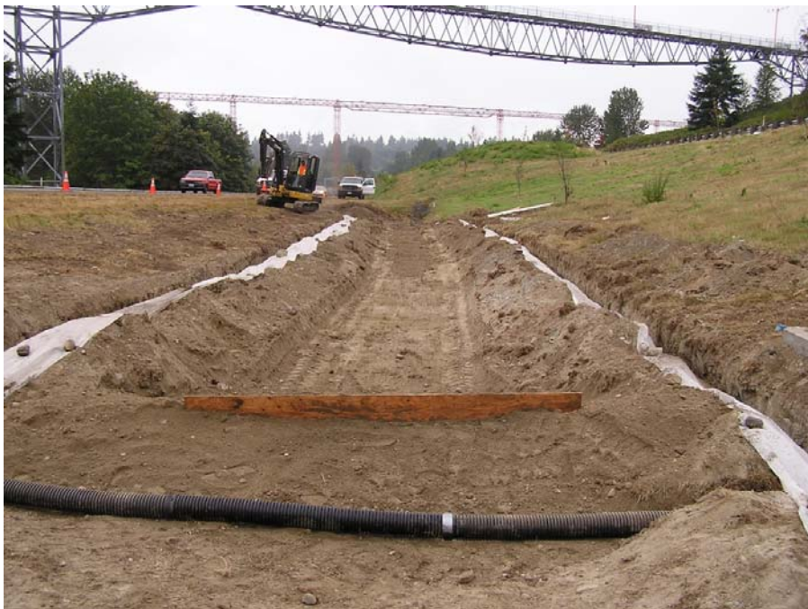
Figure 27. Bioswale 1 with dam at bottom end and French drains
