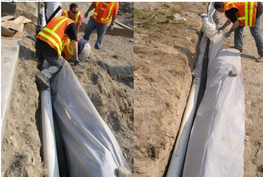
Figure 26. WSDOT workers installing pipe and plastic sheeting in French drain
