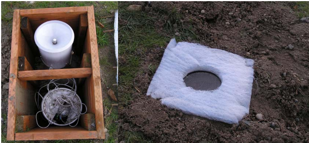
Figure 5. TB3 (left) and ISCO (right) rain gauges installed in housing in pits
