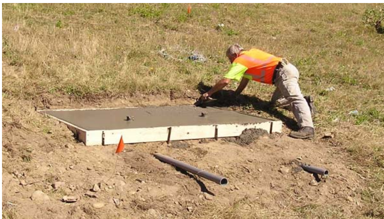
Figure 12. WSDOT employee finishing concrete pad for instrument box
