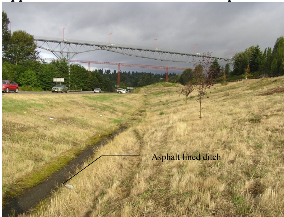
Figure 22. Bioswale site before construction began
