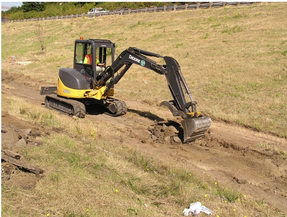
Figure 24. Excavator removing asphalt lining in ditch
