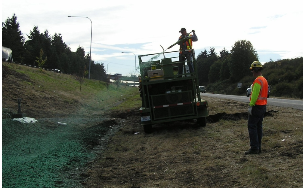
Figure 29. Bioswale with compost blanket installed
