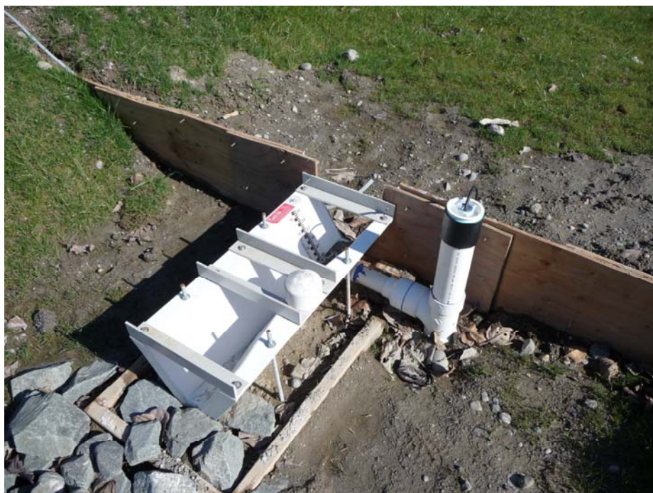
Figure 35. Parshall flume at outlet of bioswale 1
