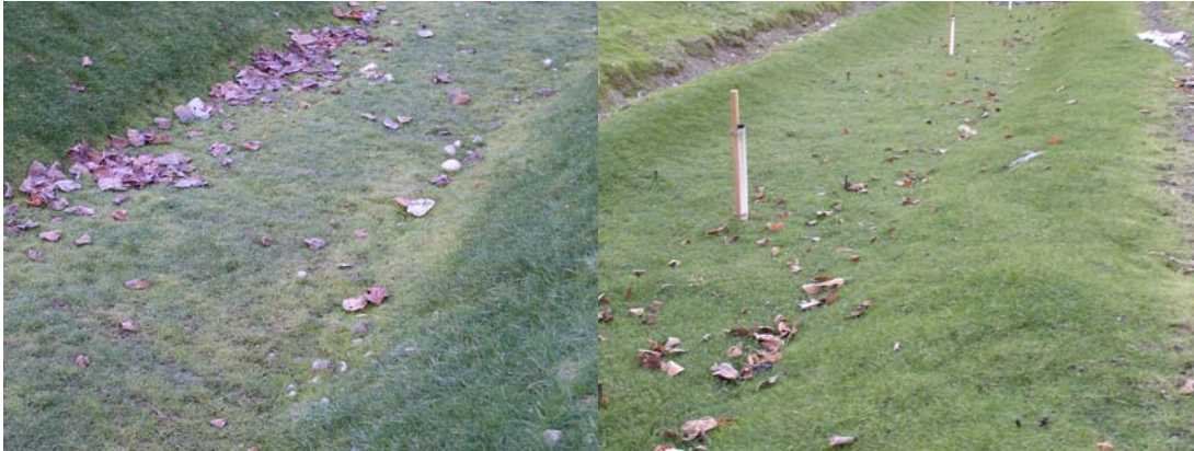
Figure 19. Bioswale 2 (left) and bioswale 1 (right)
