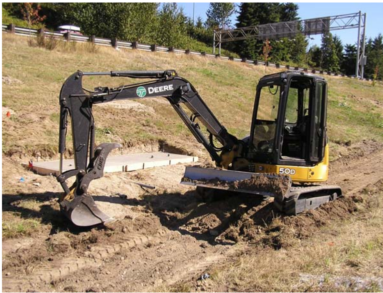
Figure 11. Excavator used to do site preparation
