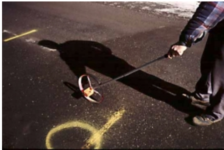
Figure 9: Measuring crack length in a surface distress survey
