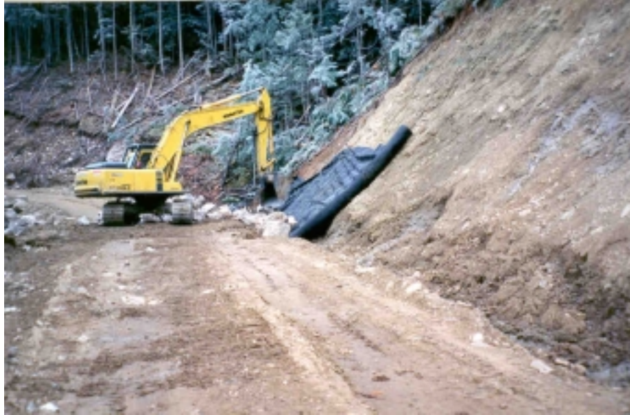
Figure 2. Placing the geotextile
