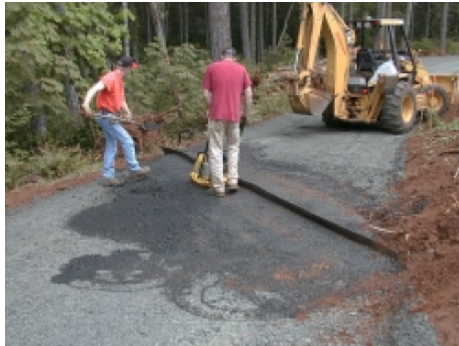
Figure 7. Installing a rubber belt cross drain on a relocated out-sloped section.
