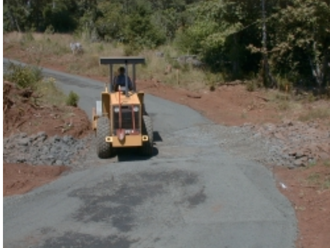
Figure 6. A ford constructed across an intermittent stream.
