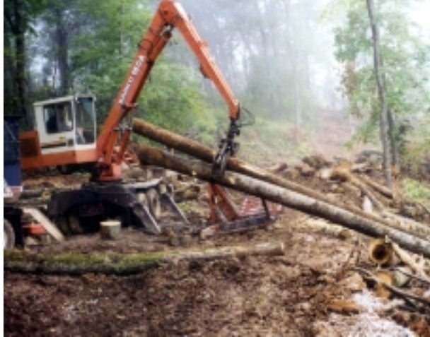
Figure 4: Poor location of the loader resulting in operational delays when loading out the truck.
