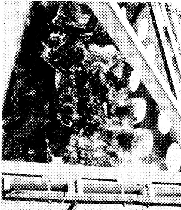
Figures 6 & 7 Breakwater Operation. (Incident wave energy converted to kinetic energy [jets] and dissipated through turbulent mixing and diffusion.)
