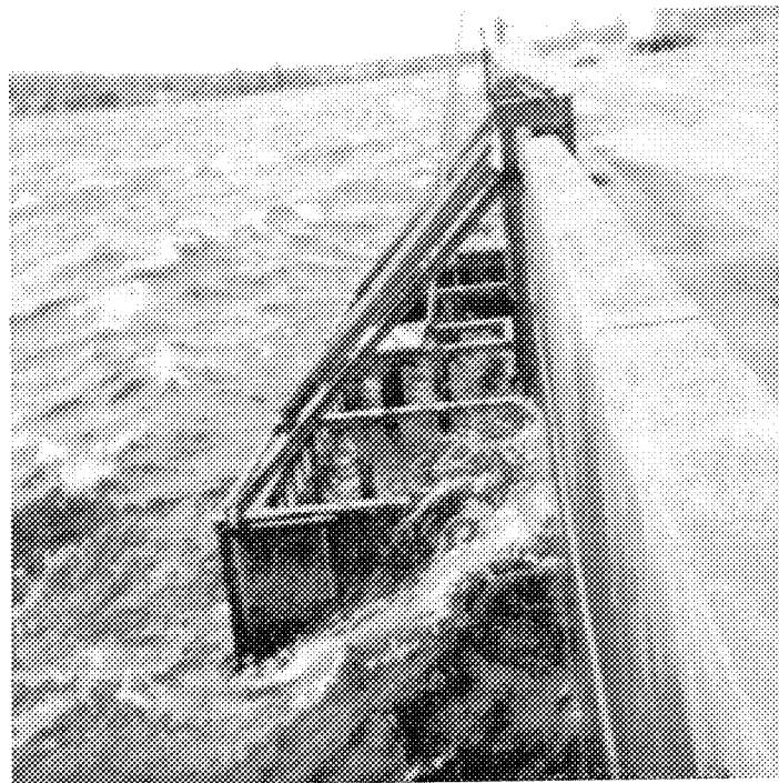
Figure 42.30-35 M.p.h. Wind Condition. Note dry roadway behind breakwater.
