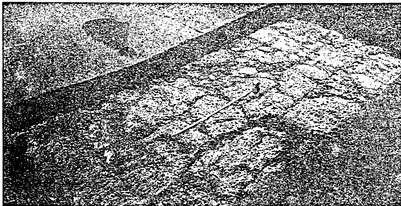
PHOTO 17.--CTB, SECTION 4 UNDER WHEEL PATHS SHOWING IRREGULAR POLYGON CHUNKS.
