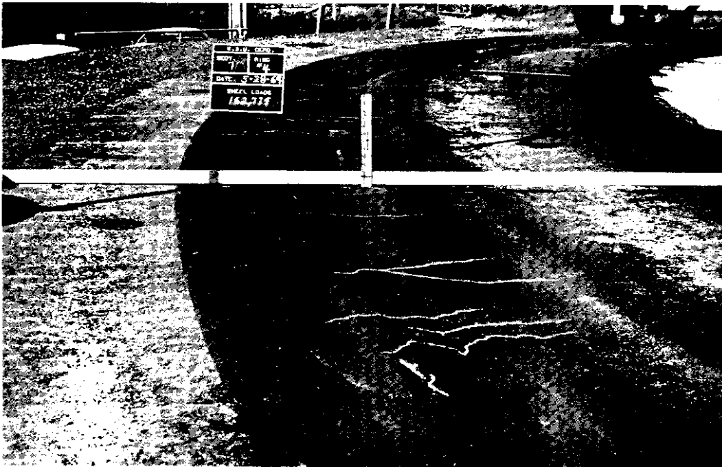
FIGURE 66. APPEARANCE OF SECTION 7 AFTER 162,774 WHEEL LOADS ON MAY 28, 1969. NOTE THE TRANSVERSE CRACKS AND THE DEPTH OF DEFORMATION.
