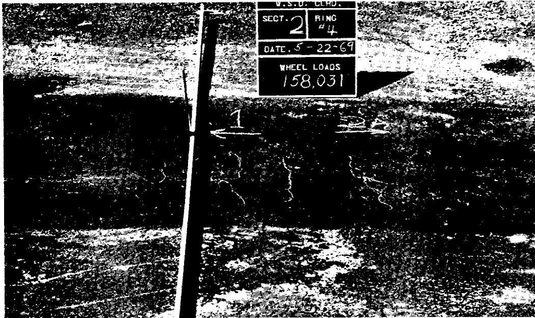
FIGURE 57. FAILURE IN THE TRANSITION ZONE BETWEEN SECTIONS 1 AND 2 AT 158,031 WHEEL LOADS--MAY 22, 1969.
