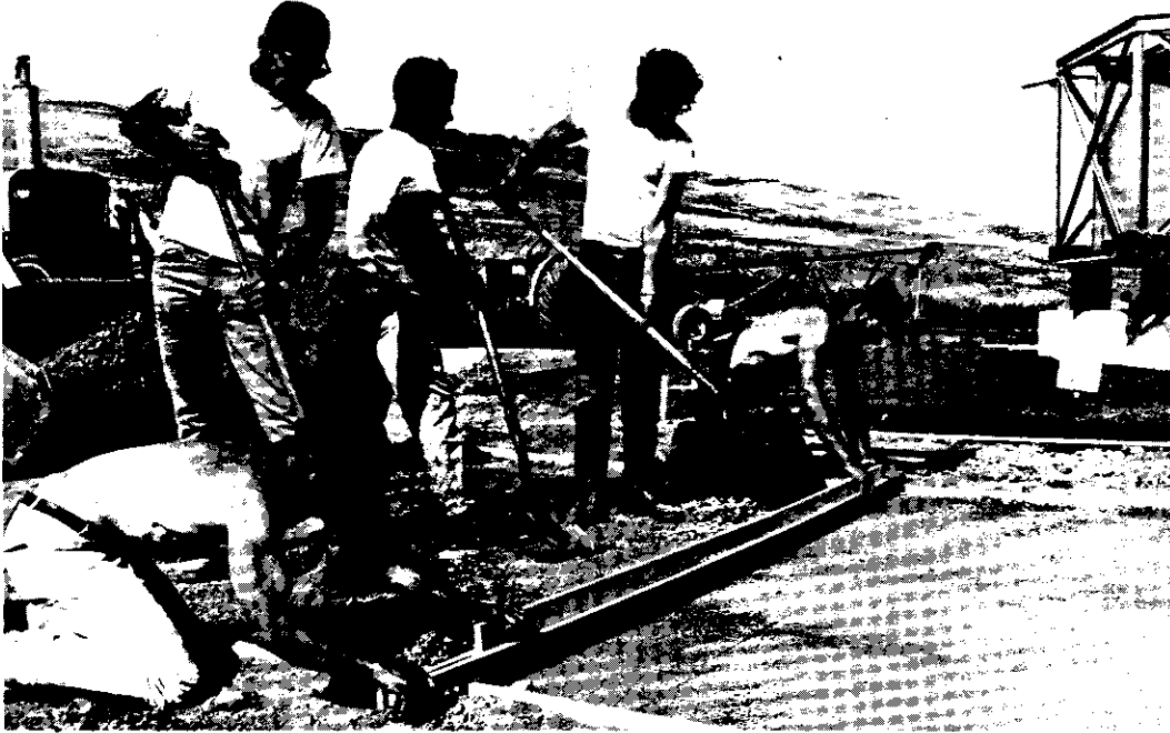
FIGURE 13. HAND WORKING AND SCREEDING OF THE SUBGRADE TO FINAL ELEVATION BY THE CONTRACTOR'S CREW. THE FORMS WERE SET TO CORRECT GRADE PRIOR TO FINAL GRADING.
