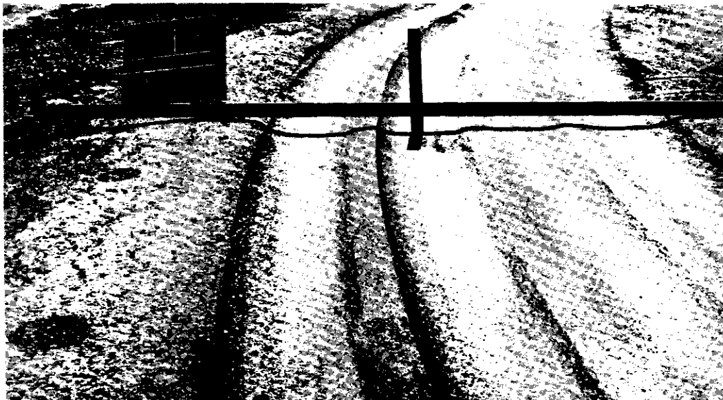
FIGURE 74. CONTINUED RUTTING OF THE ASPHALT CONCRETE OVERLAY IN SECTION 3 AFTER 211,065 WHEEL LOADS--JULY 18, 1969. NOTE DEPTH OF PAVEMENT DEFORMATION.
