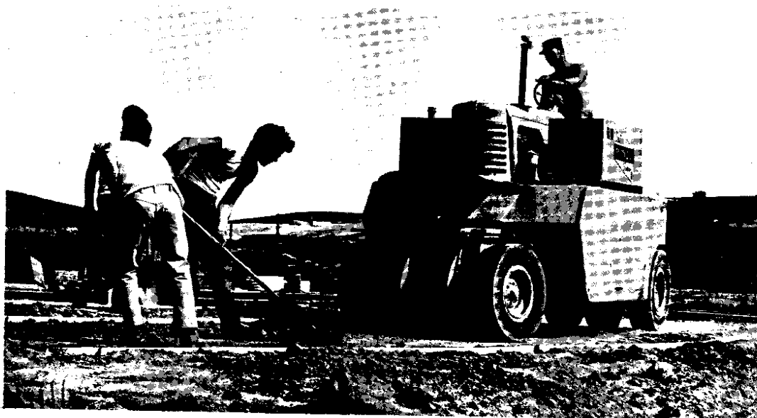
FIGURE 12. SPREADING THE SILT BY HAND AND COMPACTING WITH A PNEUMATIC RUBBER-TIRED ROLLER.
