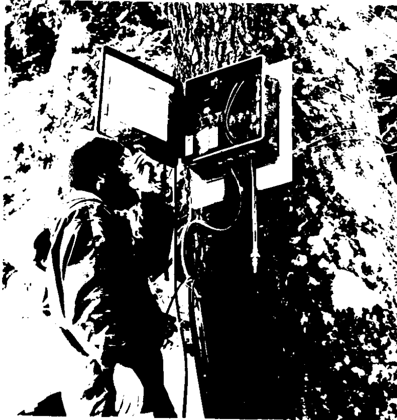
Figure 3. Gas exploder control unit installed at Old Faithful No. 7 slide path, Stevens Pass, Washington.
