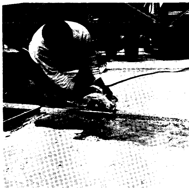
SAWING UNDERCUT OF PATCH SECTION
